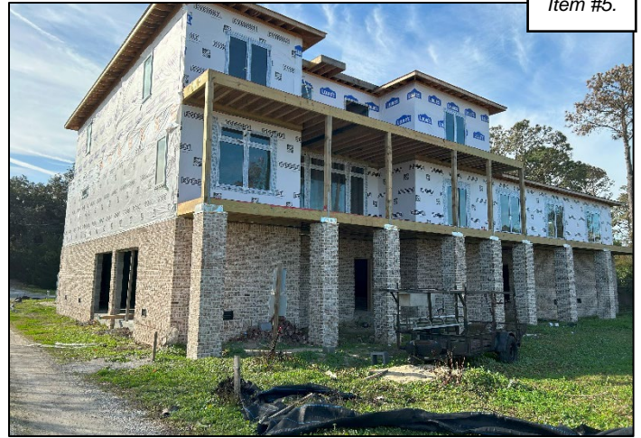
Picture 2: Existing structure
