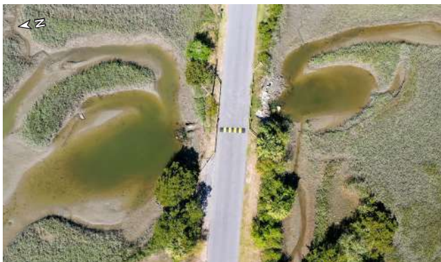
Aerial photo of the 6th St. Culvert.
