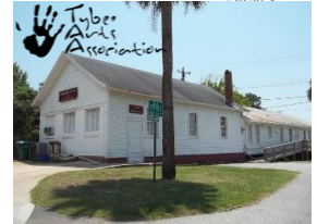
Former Ft. Screven Fire Station
