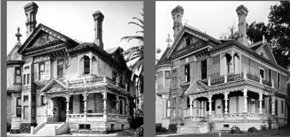
Preservation of the exterior of the Hale House, Los Angeles, California, involved repainting the exterior walls and decorative features in historically appropriate colors. An excellent example of the Preservation treatment focused upon the ongoing maintenance of historic materials and features. Photo: Before, NPS files; After: Bruce Boehner.
