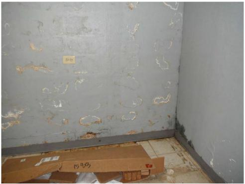
Interior - Main Building - showing mold & wall & flooring damage at SE corner of building
