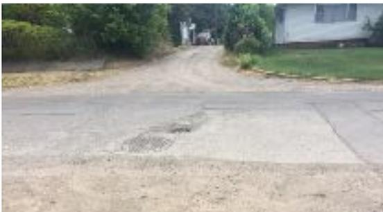
**3rd St near Minnesota Ave. showing cracking, pothole, asphalt patching and lack of storm drains, curbs and sidewalks.**
