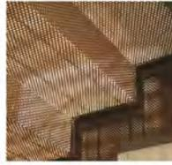
Perforated Metal Shade Panels and Backing for attachment of sign panels.
