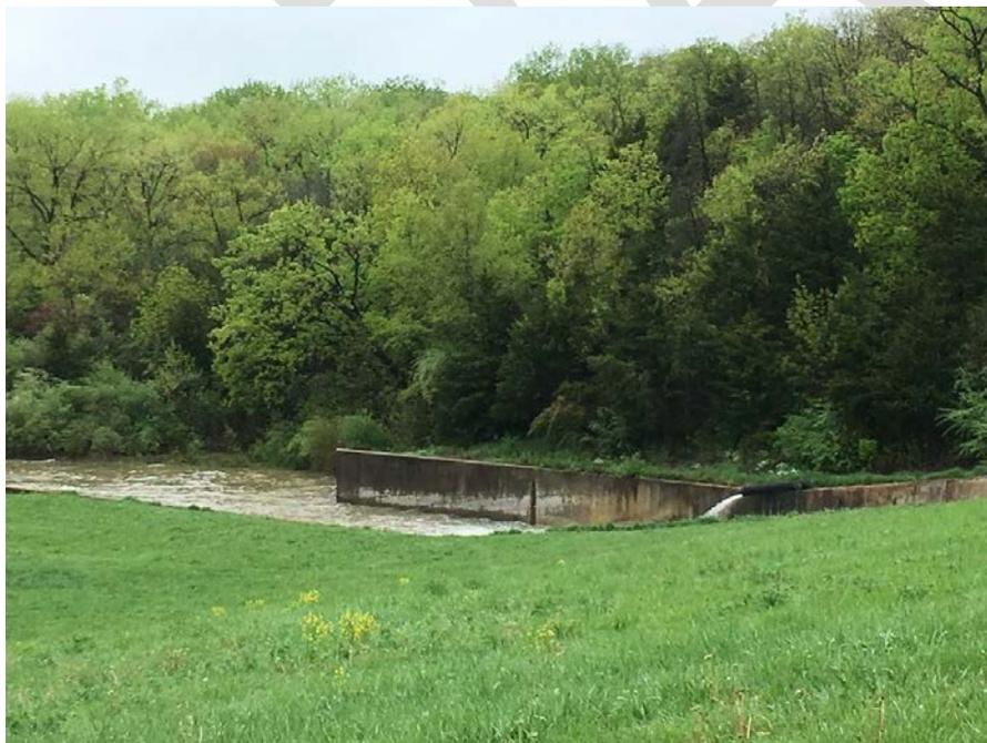
**Figure 8 Seepage Bypass from the Sugar Creek Lake Dam to the Lake Spillway**
