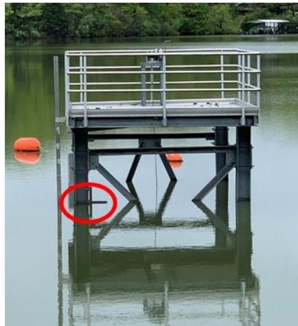
Figure 11. The City currently has to visually estimate the level of the reservoir by the use of bars (example circled) attached to the intake platform at one-foot intervals above and below normal pool.
