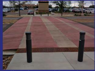
A "tabletop" pedestrian crossing which maintains the pedestrian walking surface and bollards used to separate vehicles from pedestrians.
