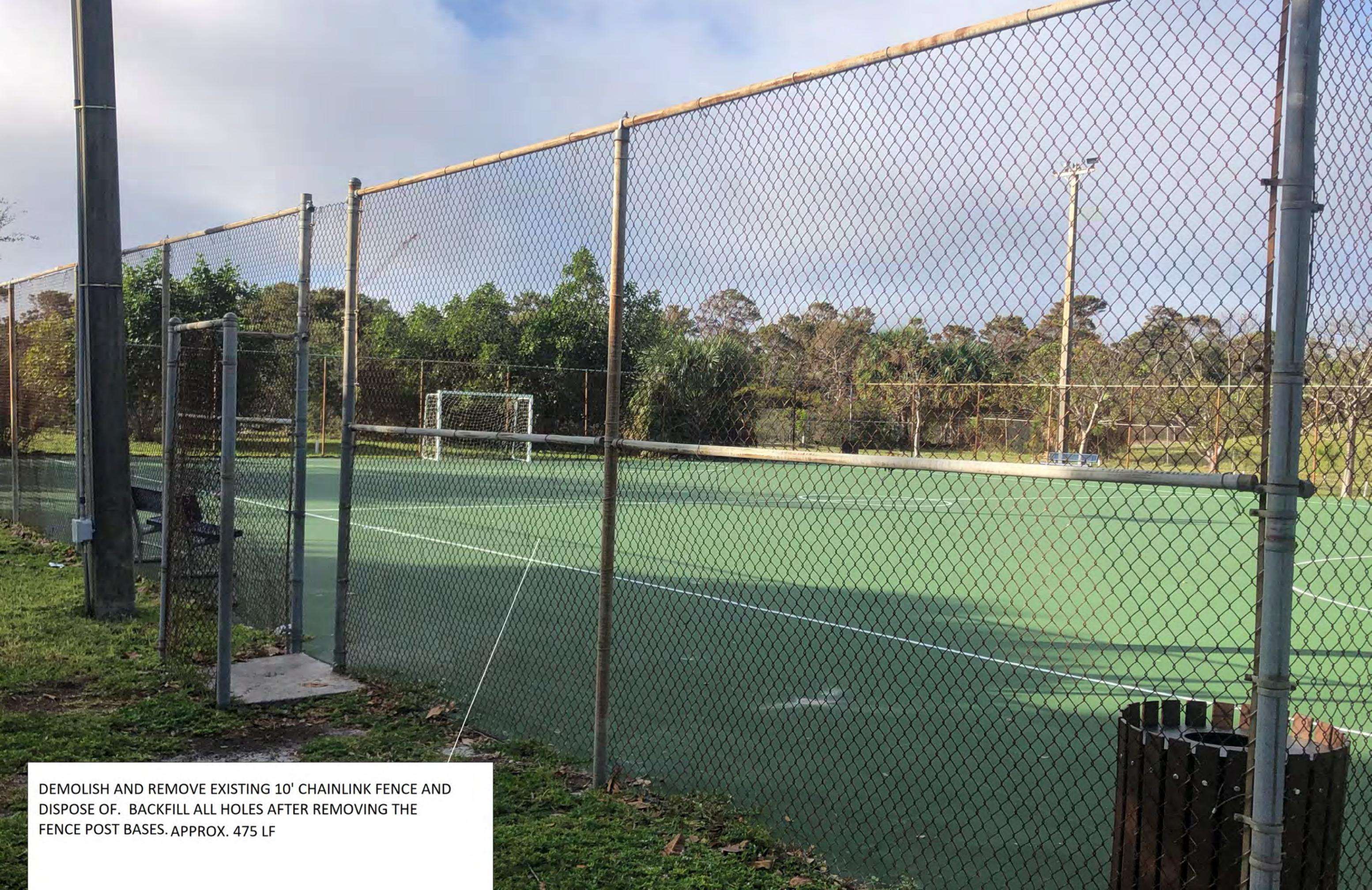
DEMOLISH AND REMOVE EXISTING 10' CHAINLINK FENCE AND DISPOSE OF. BACKFILL ALL HOLES AFTER REMOVING THE FENCE POST BASES. APPROX. 475 LF
