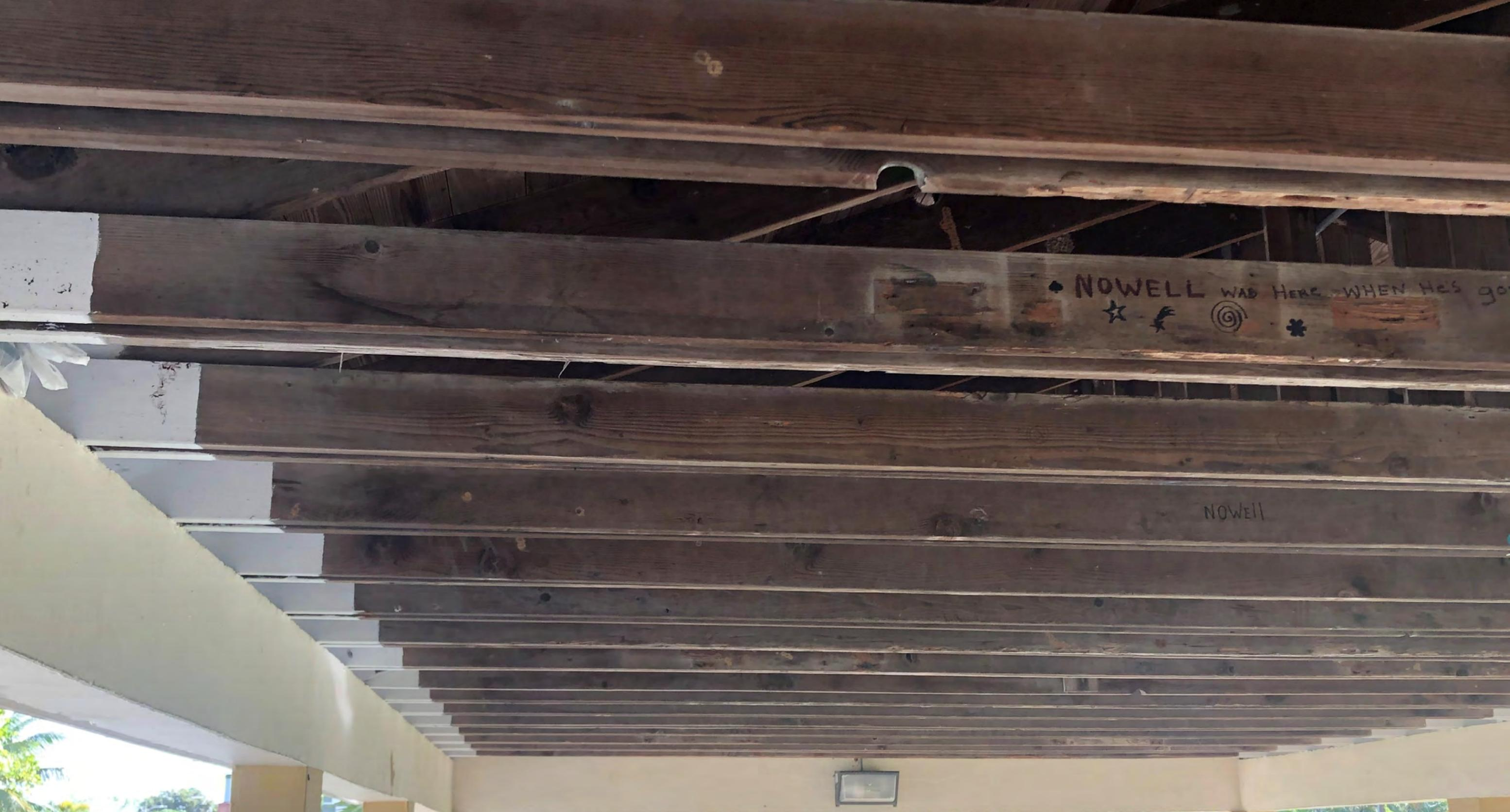
INSTALL 1/2" PLYWOOD OVER ENTIRE CEILING AREA UNDER PAVILION AND SOFFIT, LATH AND STUCCO. PAINT WITH TWO (2) COATS EXTERIOR WHITE PAINT. APPROX. 1,125 SF
