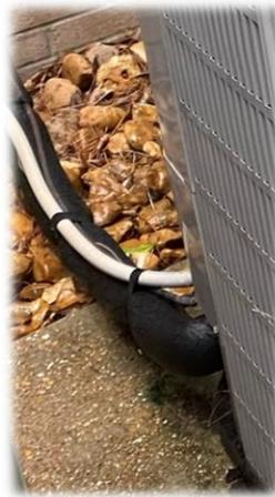
**Figure 10. Well maintained insulation on refrigerant lines at the City Hall.**
