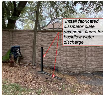
Install fabricated dissipator plate and conc. flume for backflow water discharge
