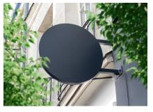
Projecting Nameplate Sign. A sign affixed to any party of a building or structure which extends beyond the building or structure by more than 10 inches. A SIGN indicating only the name and/or address of a business or occupant(s) that extends outward, perpendicular to the BUILDING face, not more than four feet (4') beyond the BUILDING and not less than eight feet (8') above the sidewalk or ground level.
