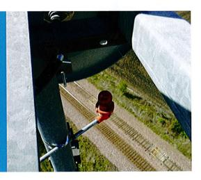
supported by a top appurtenance. For example, the beacon can be mounted on a pole (the pole should be designed for this intent and certified to the TIA-222-G addendum II specification) and raised above an array of panel antennas. If raising the beacon would prohibit future inspection and maintenance, the beacon may be lowered to a maximum of 10' below the top of any antenna or
