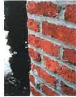
Abrasive cleaning can cause permanent damage to historic fabric, such as this brick wall. Photo: NPS files.
