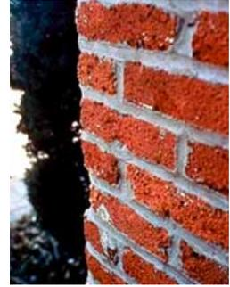
Abrasive cleaning can cause permanent damage to historic fabric, such as this brick wall. Photo: NPS files.
