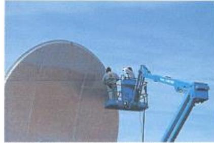
Soda blasting a radio dish at Hat Creek Radio Observatory
