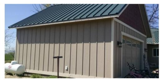
Garage roof and siding to be composed of steel standing seam (above) or similar approved metal panel product (per zoning code and variance conditions, corrugated metal is **not** an approved material and will not be used). The roof will be red and the siding will be white/offwhite, matching the existing red shingles and off-white stucco on the house as close as possible. Image retrieved from http://go-rsp.com/panels/panels/sl-15-standing-seam/
