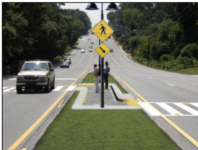
*A gap and channelization in this raised median places pedestrians in correct orientation to cross*
