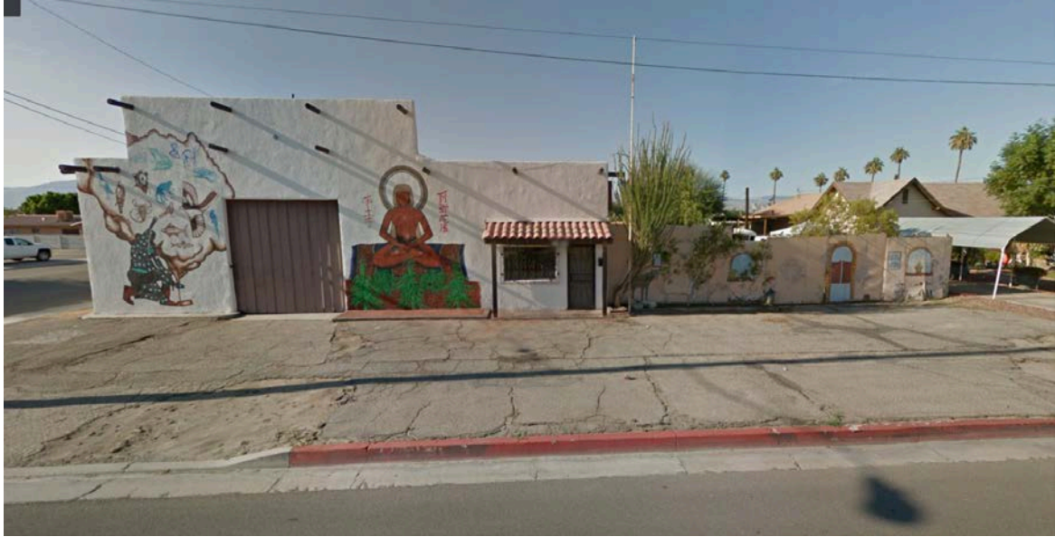
The photograph below shows the exterior elevation of the building along the Third Street frontage as it looked in November, 2018.
