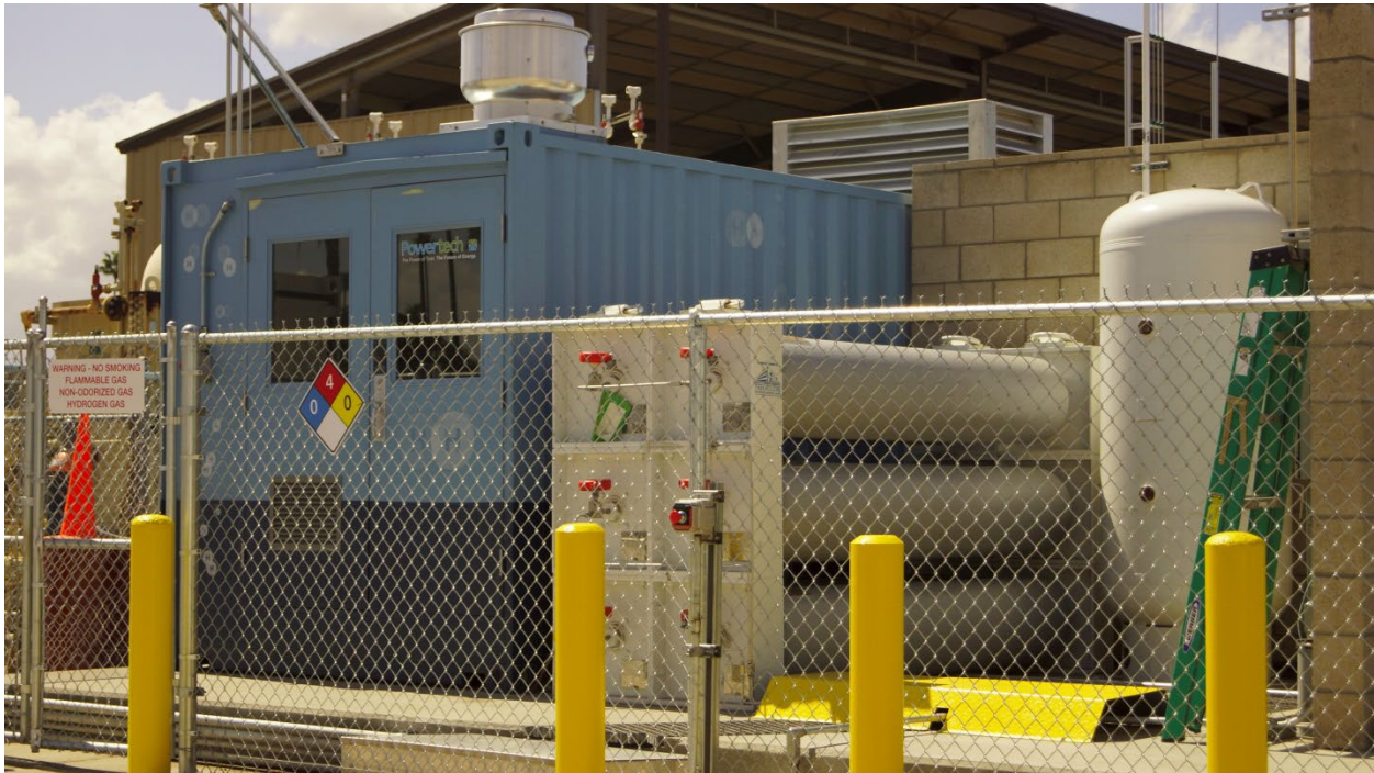
Figure 1: Powertech fuel processing module and high-pressure storage at the Riverside hydrogen refueling station. Image Credit: Hydrogen Ventures.
