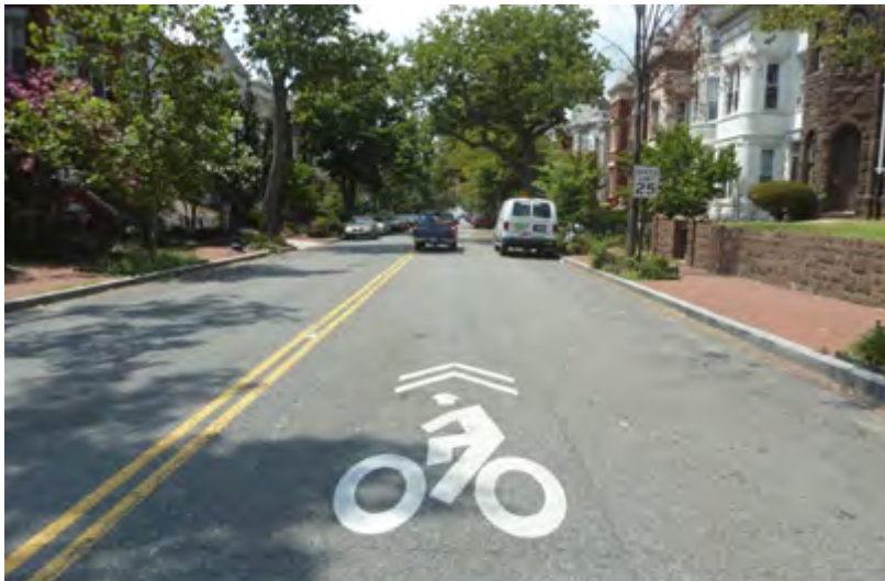
Figure 69: Example of shared lane markings used on bike boulevard (Class III bike route)
