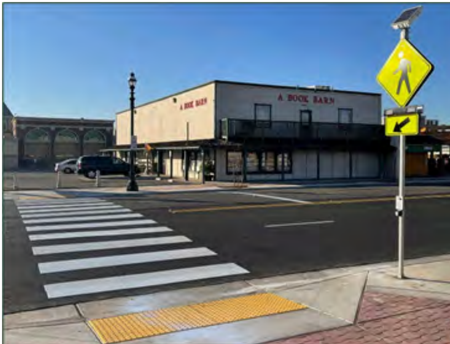
Figure 27: Rectangular Rapid Flashing Beacon (RRFB)
