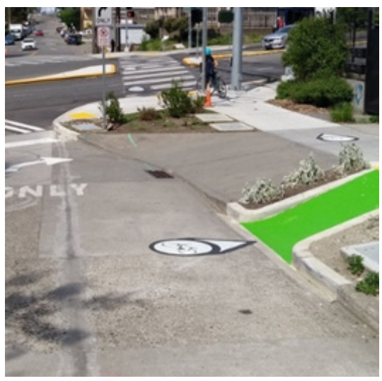
Figure 70: Example of a bike wayfinding dots used to guide users through an intersection
