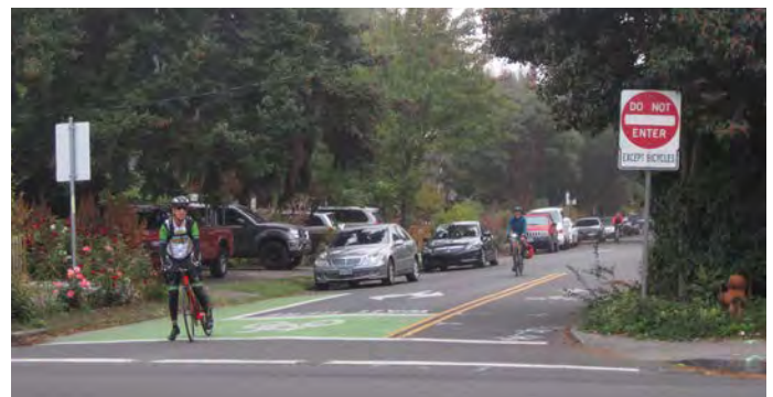
Figure 46: Bicycle Box with Lead-In Bike Lane
