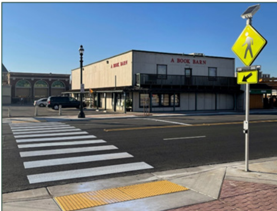
Figure 27: Rectangular Rapid Flashing Beacon (RRFB)
