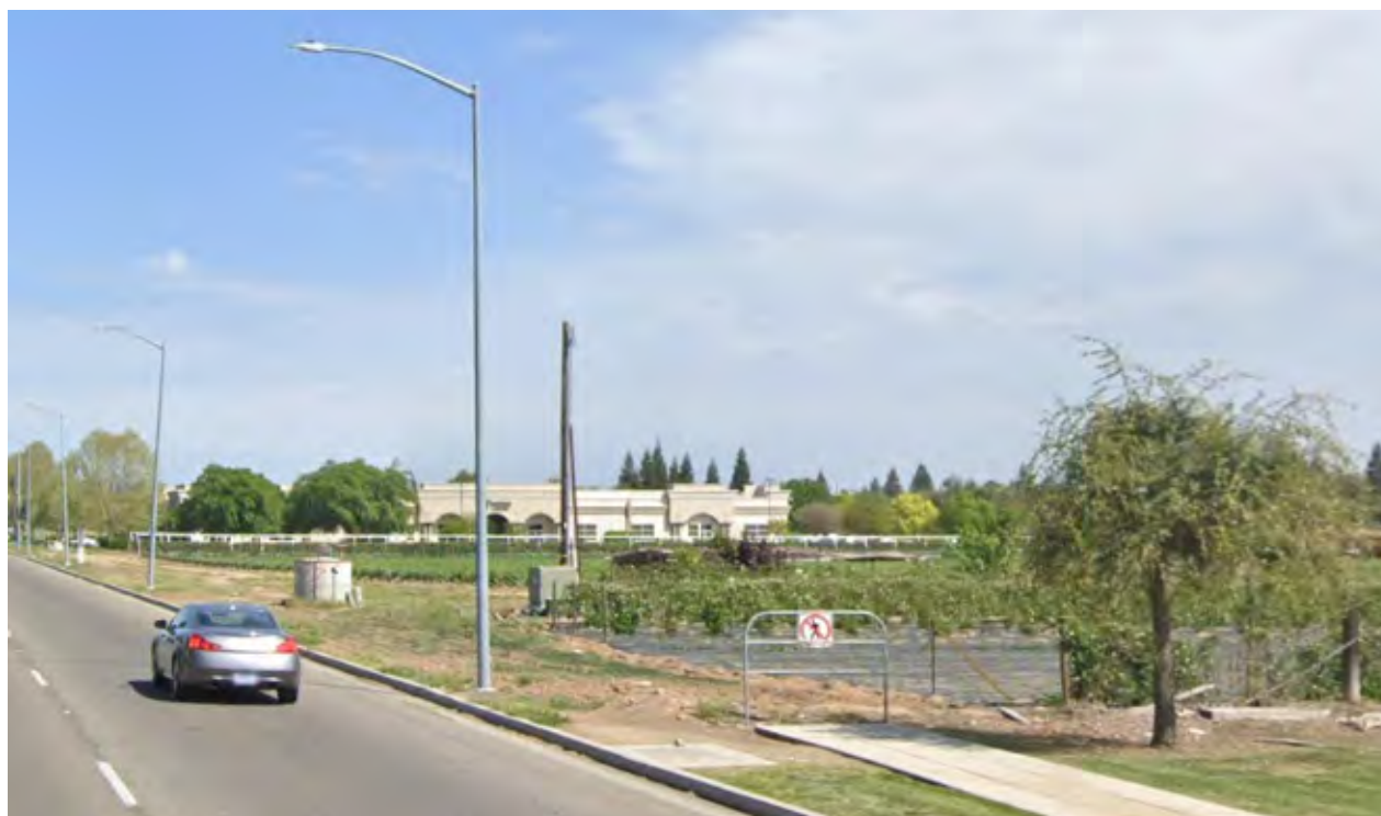
Figure 4: There is a Gap in the Sidewalk Network on the South Side of East Herndon Avenue between North Willow Avenue and North Peach Avenue
