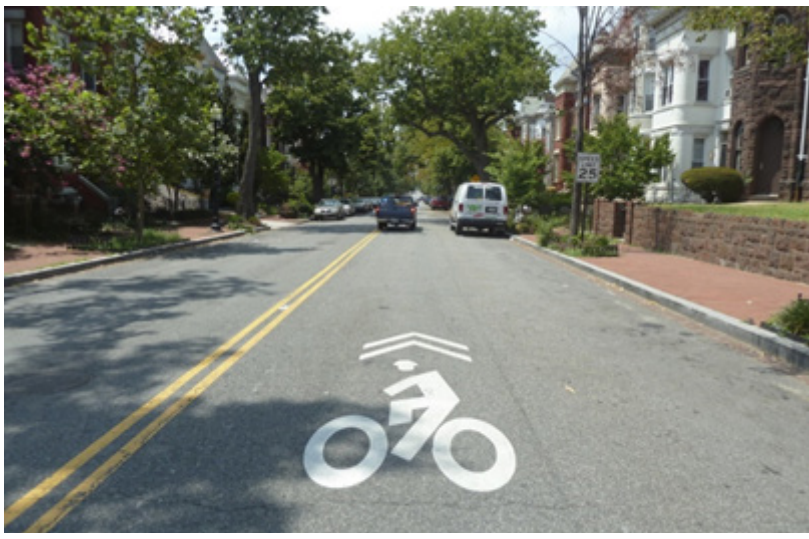
Figure 69: Example of shared lane markings used on bike boulevard (Class III bike route)
