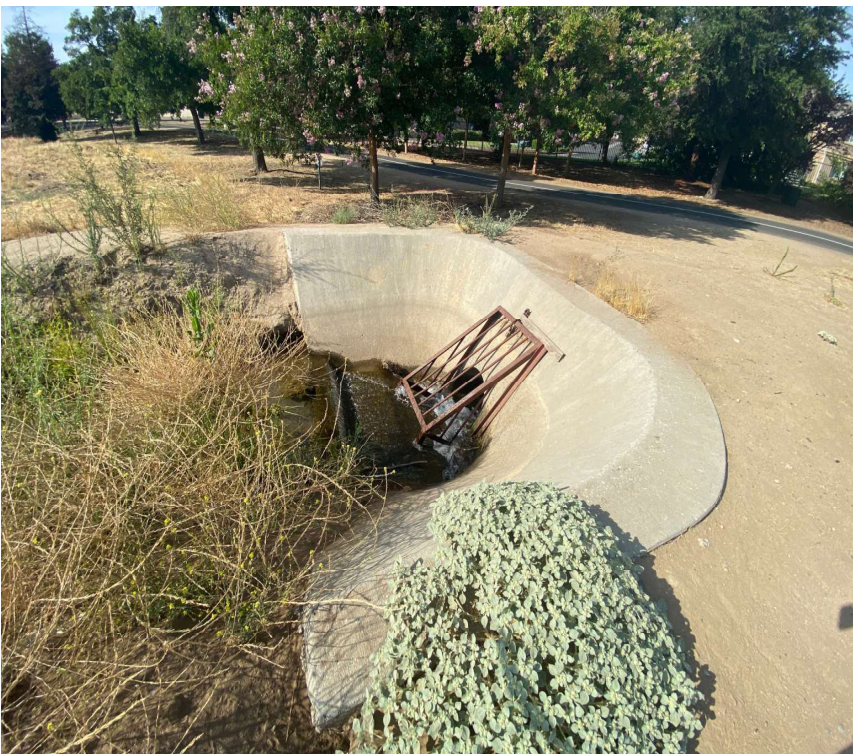
Photograph 4: Western end of ditch with concrete apron where water re-enters the subsurface pipe, looking southwest.
