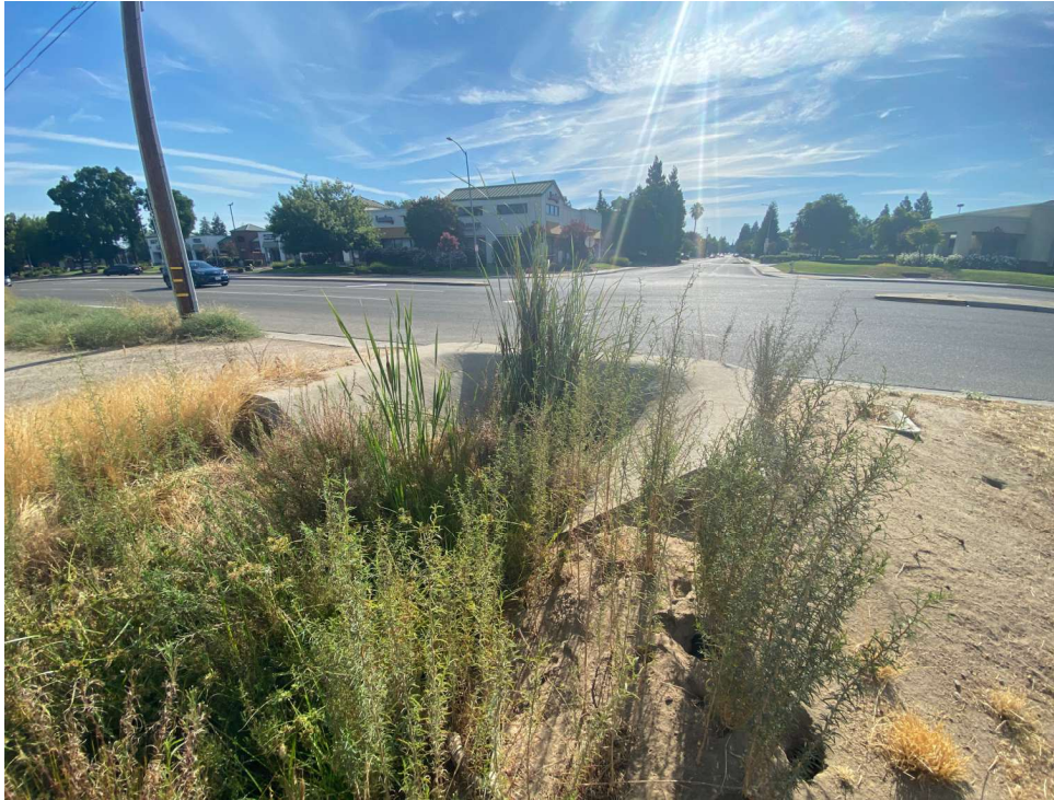
Photograph 1: Eastern end of ditch and concrete apron where the conveyance daylights. View east with N. Clovis Avenue (mid-ground) and Palo Alto Avenue (background) visible.
