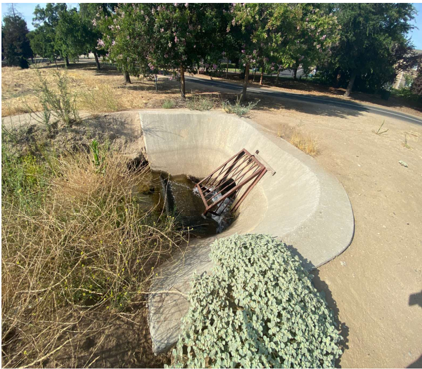
Photograph 4: Western end of ditch with concrete apron where water re-enters the subsurface pipe, looking southwest.
