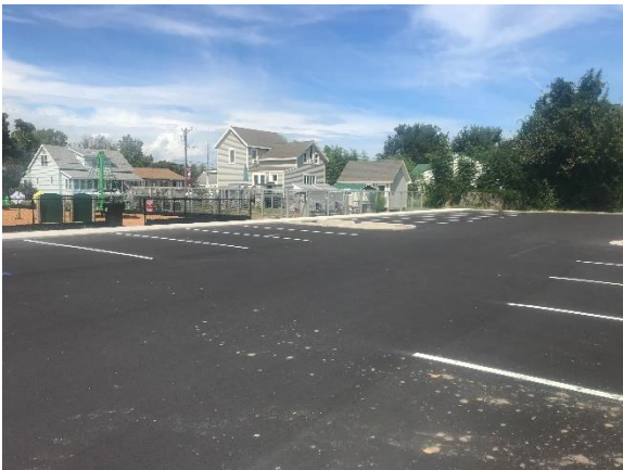
Completed parking lot striping using pre-cut thermo plastic
