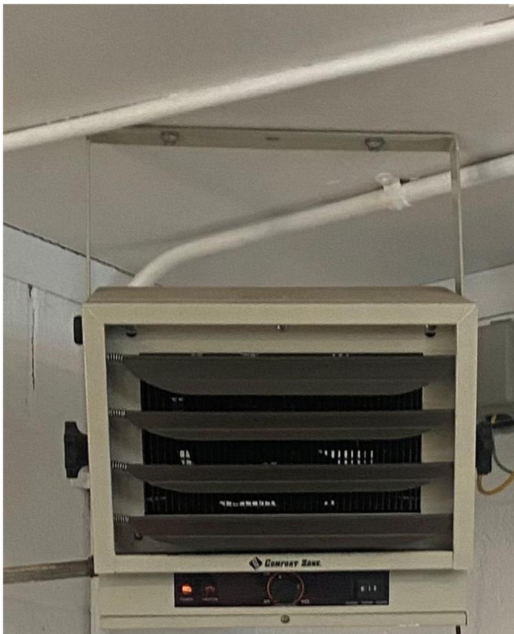
Heater was replaced in Well 6 building.
