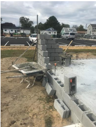
Began erection of block walls
