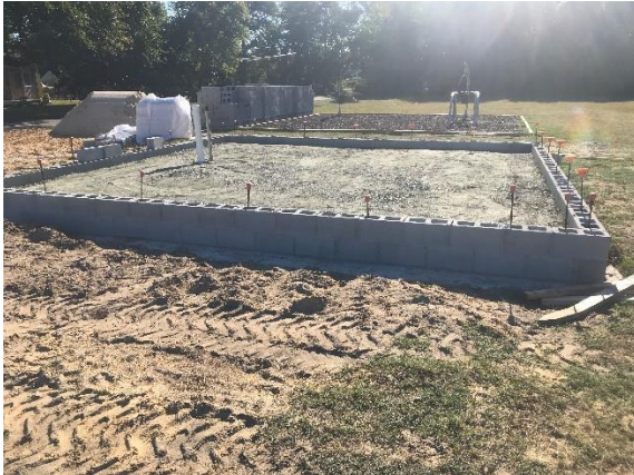
Backfilled and tamped restroom foundation
