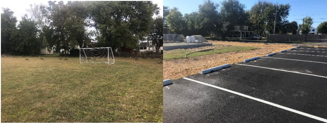
Assembled and temporarily placed soccer goals Placed parking bumpers
