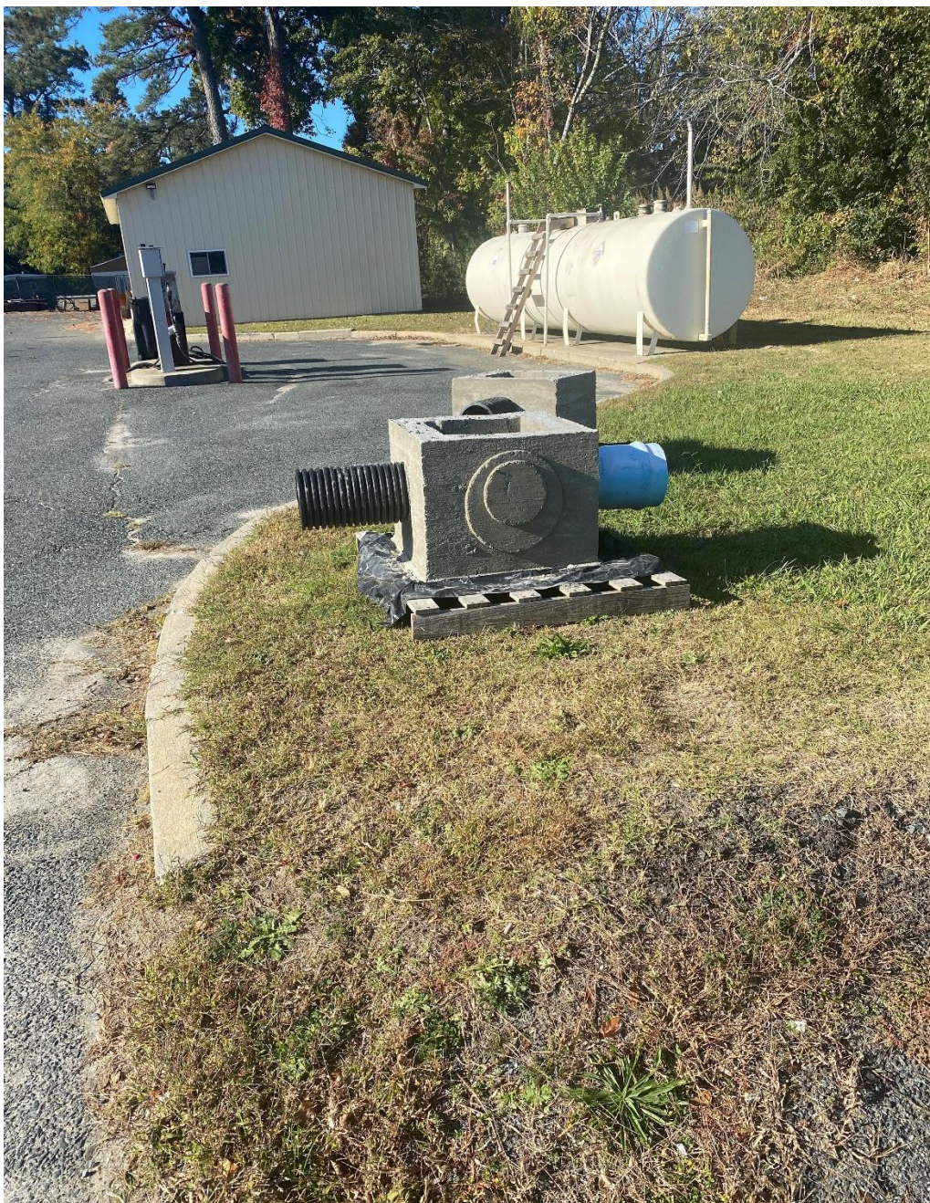
Inlets were made in preparation for stope drain replacement on Poplar Street.
