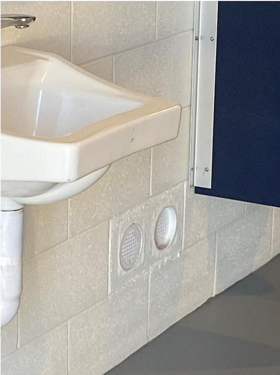
New vents installed after vandalism at Brianna's Park.
