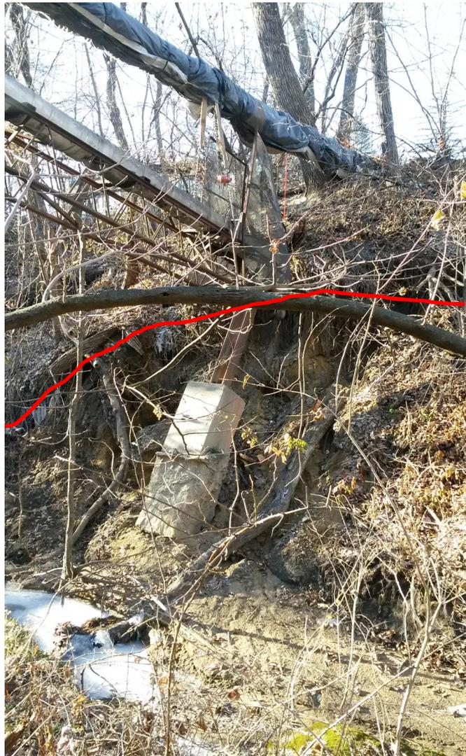
Figure 1. West ravine slope failure with scarp marked in red
