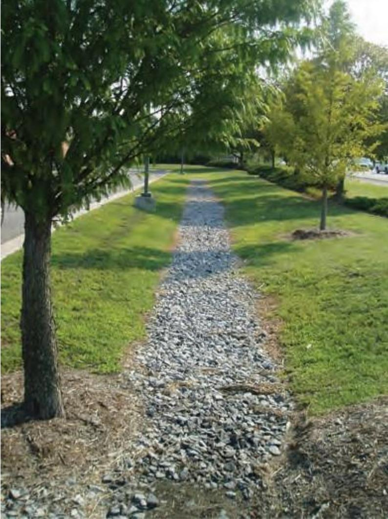
Figure 4.16. Infiltration practice in median strip.
