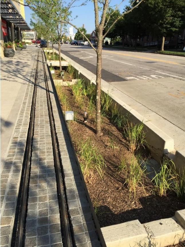
Figure 4.5. Example streetscape bioretention.
