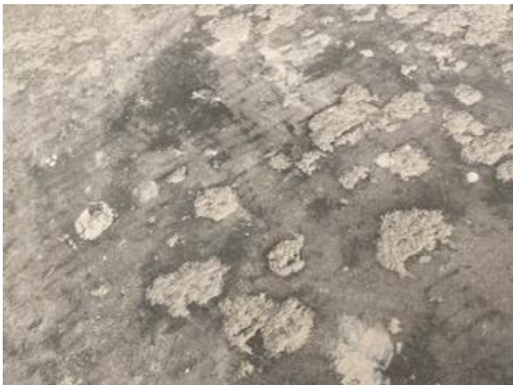
FLOOR EPOXY DAMAGE
