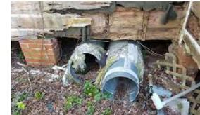
Figure 46. Missing Packaged HVAC System
