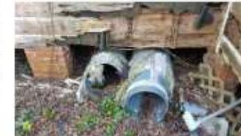
Figure 46. Missing Packaged HVAC System
