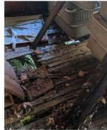
Figure 54. Flooring deterioration in NW bedroom
