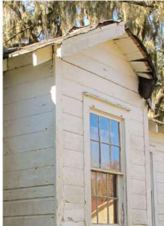
Figure 13. Barge rafters missing at bathroom extension
