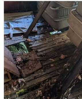
Figure 54. Flooring deterioration in NW bedroom
