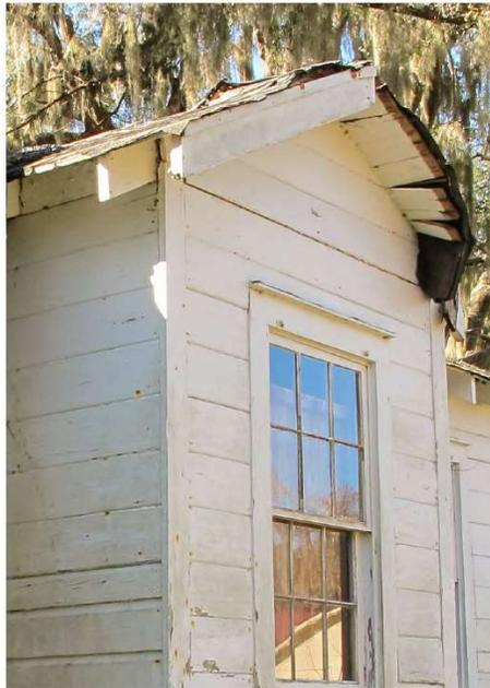
Figure 13. Barge rafters missing at bathroom extension
