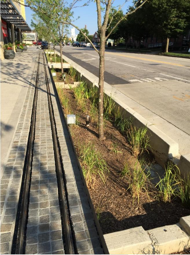
Figure 4.5. Example streetscape bioretention.
