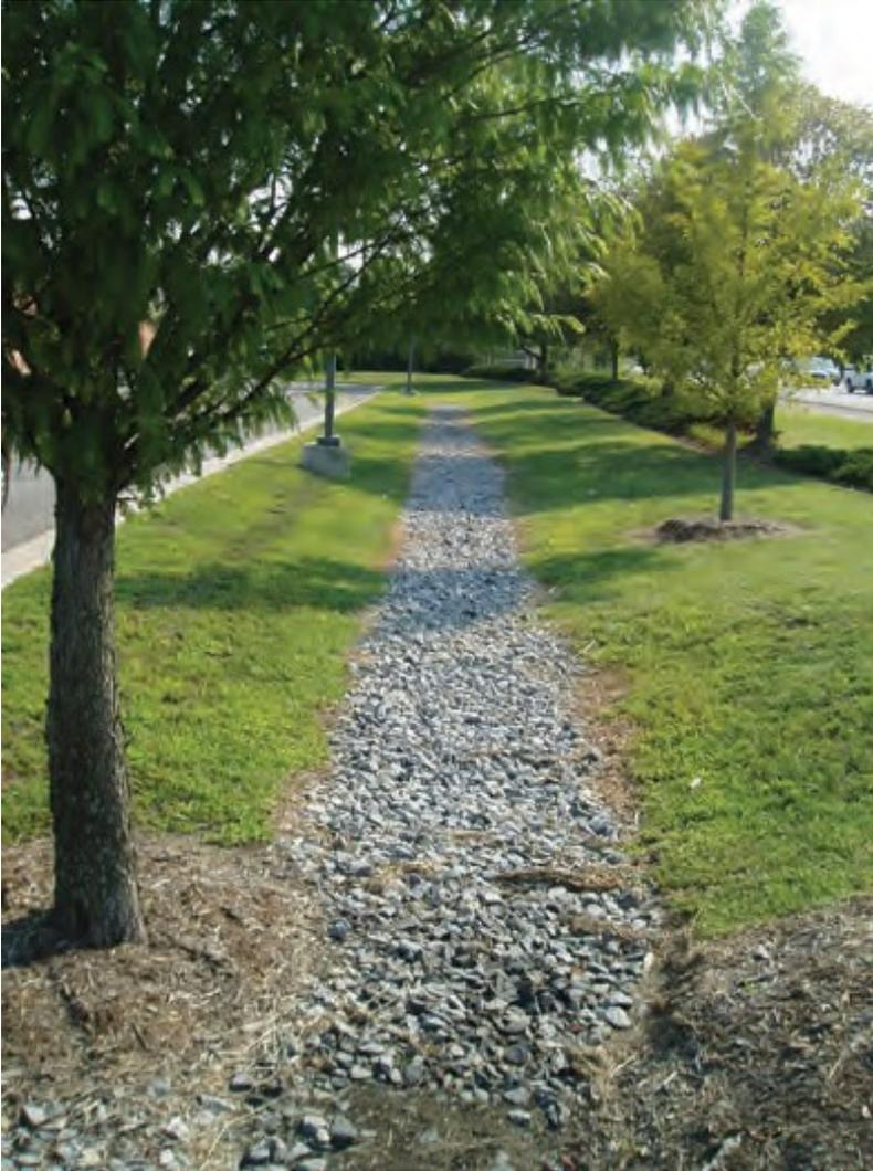
Figure 4.16. Infiltration practice in median strip.
