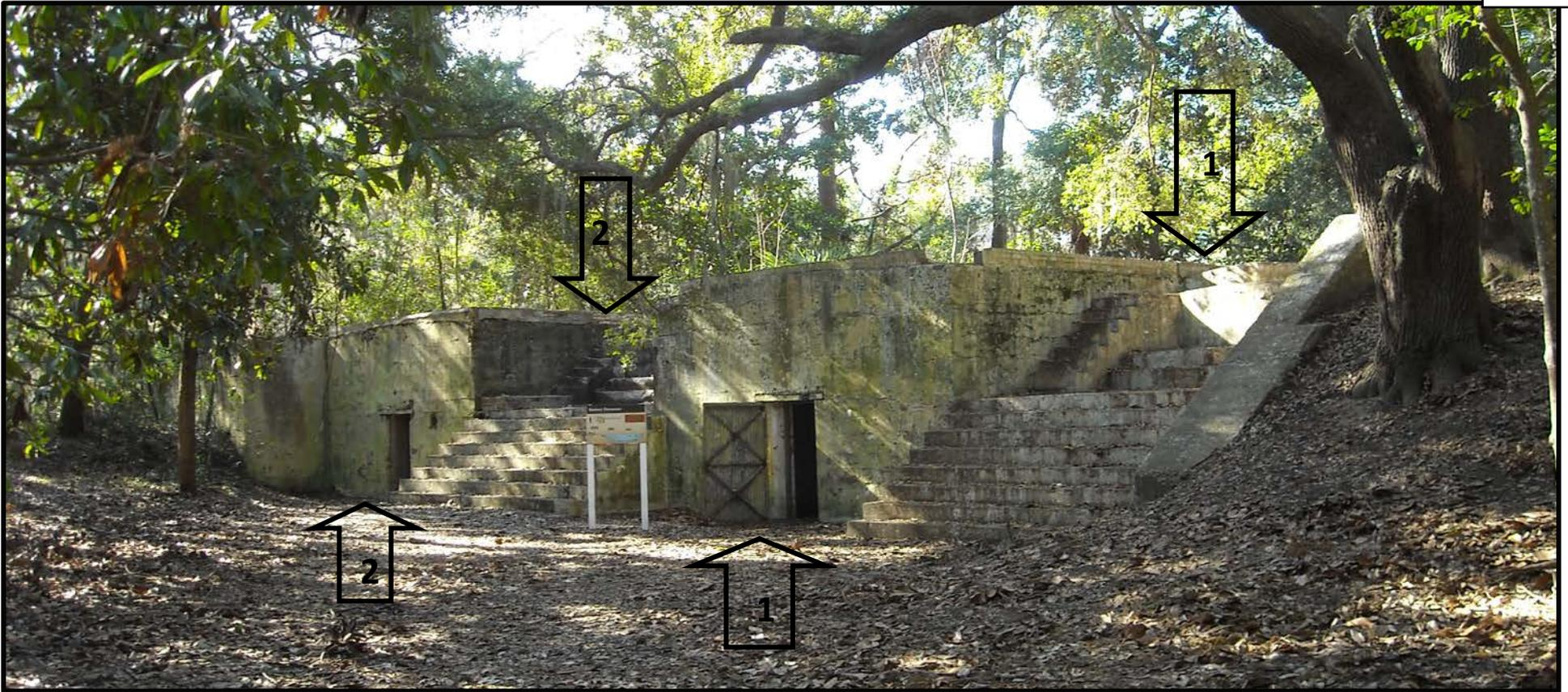
The rear of battery Fornance. The two down arrows point to the two gun positions; #1 gun on the right and #2 gun on the left. The up arrows point to the two magazines; on the right is the #1 gun magazine and on the left is gun #2 magazine.
