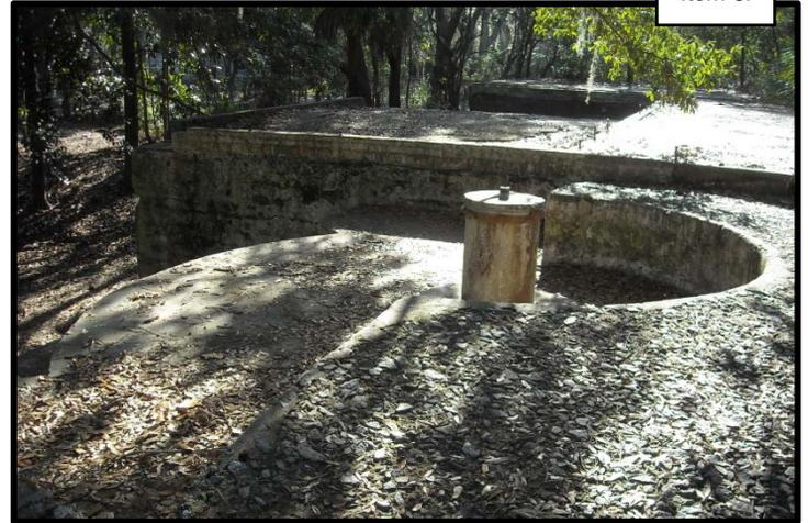
The parapet of Battery Fornance at gun #1. Left is looking north toward Battery Jesup, the right is looking south toward the #2 gun position at Battery Fornance. The large concrete column in the center is the pedestal on which the 4.72-inch gun was mounted.
