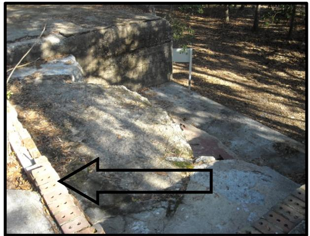
Battery Fornance #2 gun position. (Left) This is looking north toward the traverse and gun #1 position. (Right) This is a detail of the #2 gun position. The arrow is pointing to a low course of bricks that surrounded the gun position. The concrete pedestal was removed. The few bricks are the only remnants of the house that was constructed on top of the #2 gun position.
