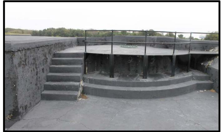
(Left) The rear of Battery Fornance #1 gun position, note the stairs up to the gun position. (Right) The iron and steel loading platform, which was removed at Battery Fornance for scrap, probably during WW II. This existing platform is at Battery Bingham, a similar 4.72-inch battery at Fort Moultrie, Sullivan's Island, SC.
