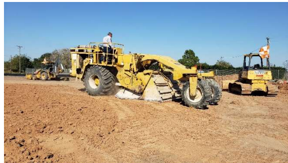
Figure 4 - Select fill mixing on the building foundation
