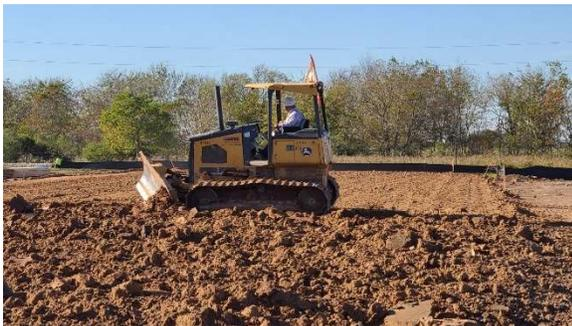
Figure 3- Folding Sand into Existing Fill
