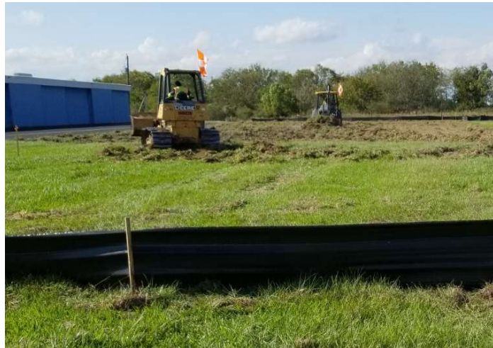
Figure 2 - Stripping topsoil for grading
