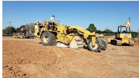
Figure 4 - Select fill mixing on the building foundation
