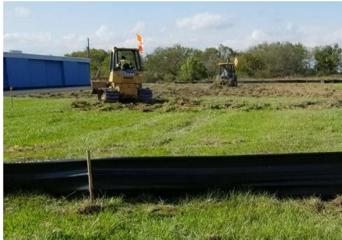
Figure 2 - Stripping topsoil for grading
