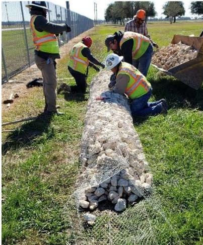
Figure 1- Installation of Filter Dam
