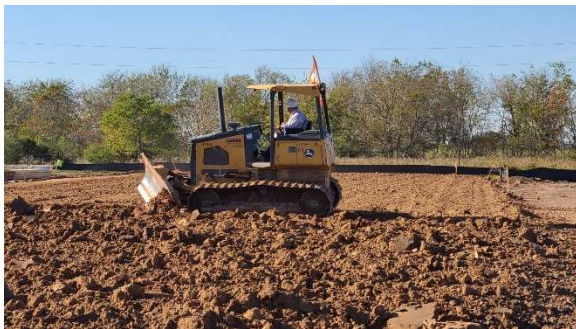
Figure 3- Folding Sand into Existing Fill
