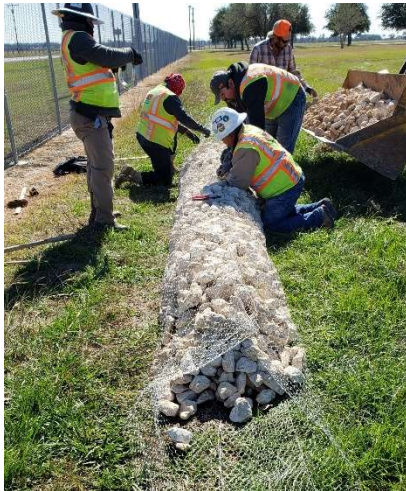
Figure 1- Installation of Filter Dam
