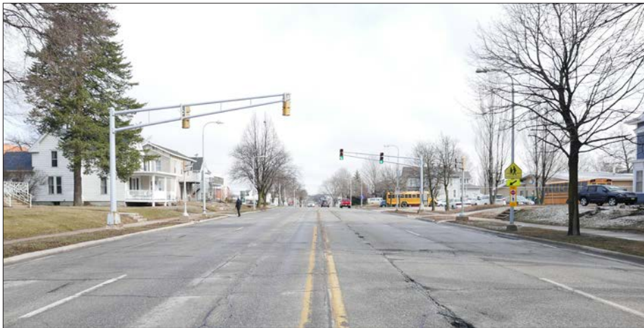
Current view looking north up Main Street toward 7th Street.
