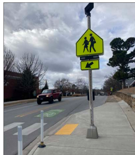
Rectangular Rapid Flashing Beacon
