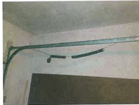
Damaged spring/cable
