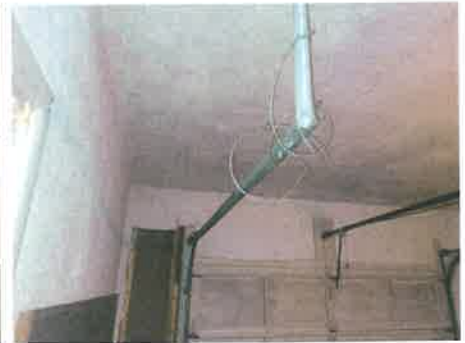
Missing spring/cable
