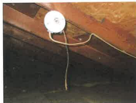
Attic--abandoned wiring
