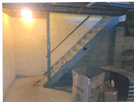
Missing guardrail
