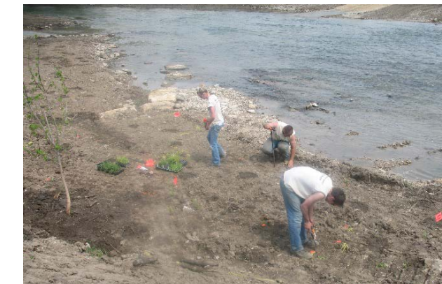
Photo 46. Planting vegetative plugs. Source: Iowa DNR
