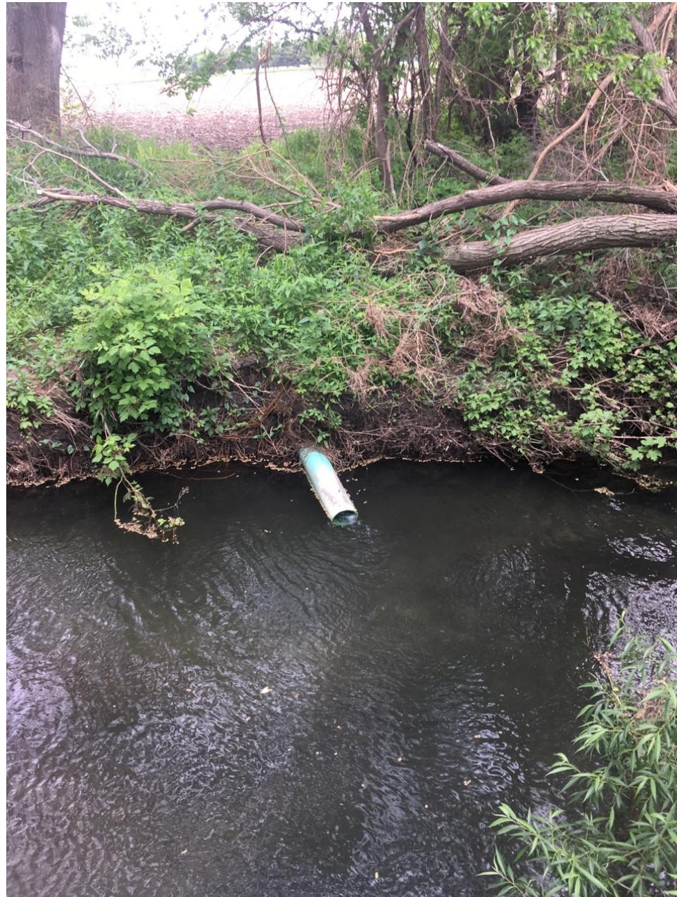
Figure 7. Pool below tile drain outfall.
