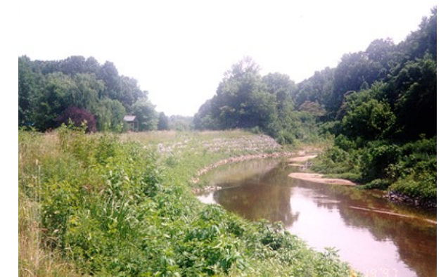
Photo 8. Joint planting with new growth. Source: Charlotte-Mecklenburg Storm Water Services
