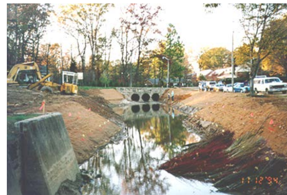
Photo 15. Cuttings stored in water before made into fascines. Source: Charlotte-Mecklenburg Storm Water Services
