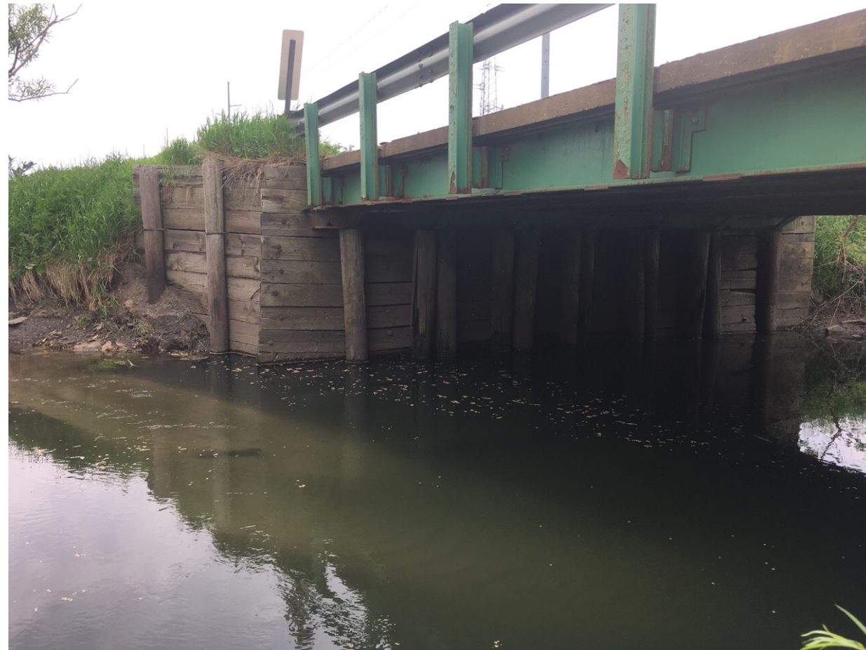
Figure 12. Stream diversion and scour pool upstream of the Ridgeway Avenue bridge.
