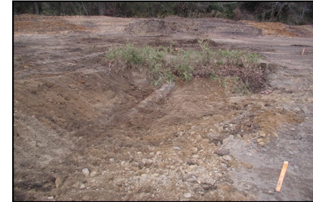
Photo 32. Sod mat placed to form stream bank. Source: Buck Engineering
