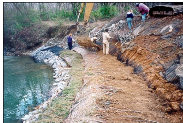
Photo 23. Bench excavation for brush layering. Source: Stantec
