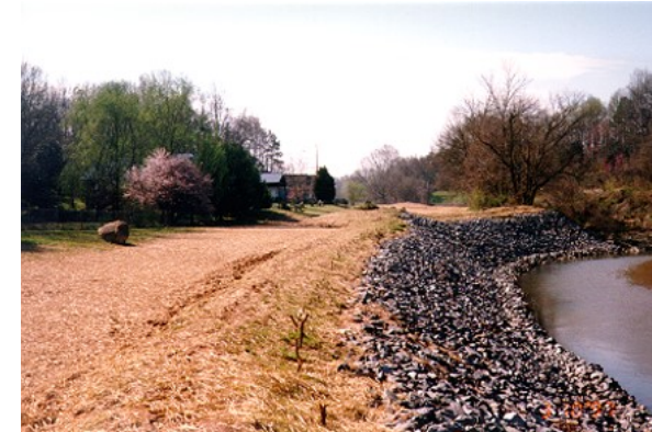
Photo 7. Joint planting. Source: Charlotte-Mecklenburg Storm Water Services
