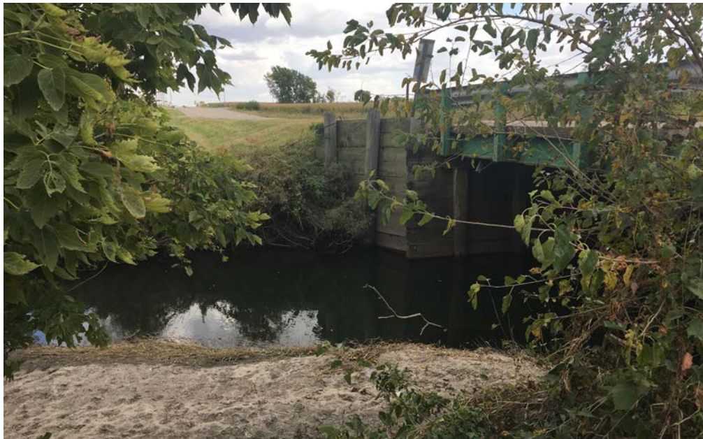
Ridgeview Ave Bridge crossing at Dry Run Creek
