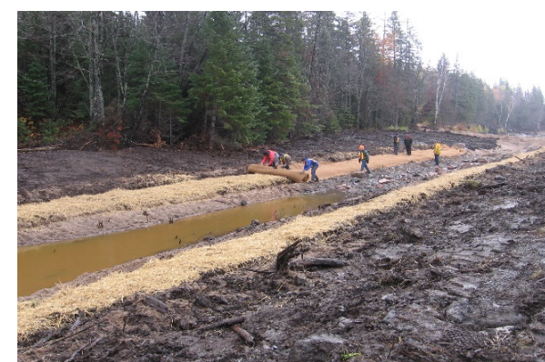
Photo 30. Erosion control matting being rolled onto a stream bank. Source: Collins & Baker Engineering
