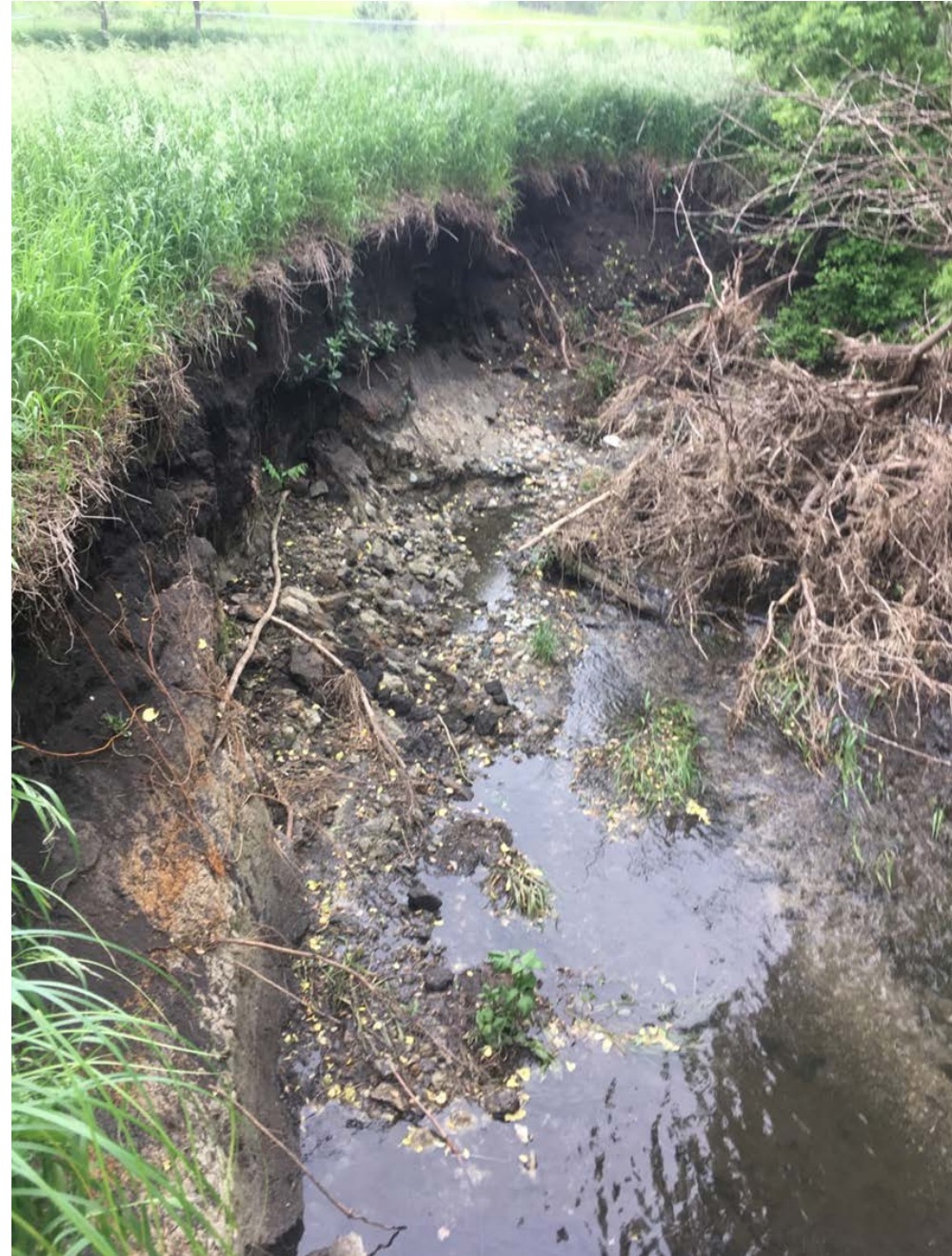
Figure 8. Typical four- to eight- foot stream bank incision within project reach.
