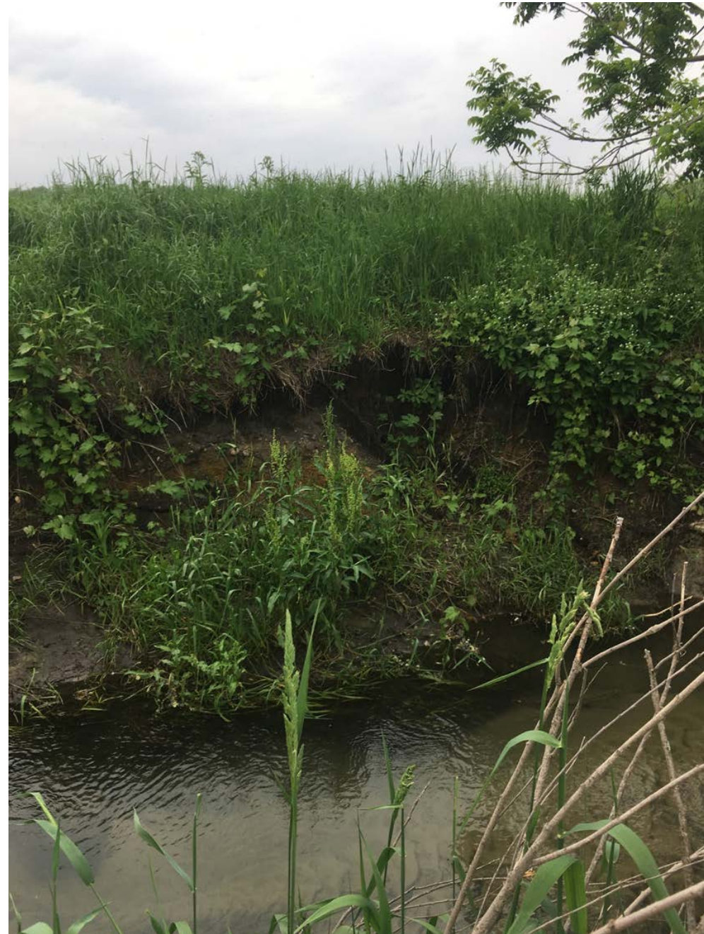
Figure 10. Example slumping of banks within project reach.
