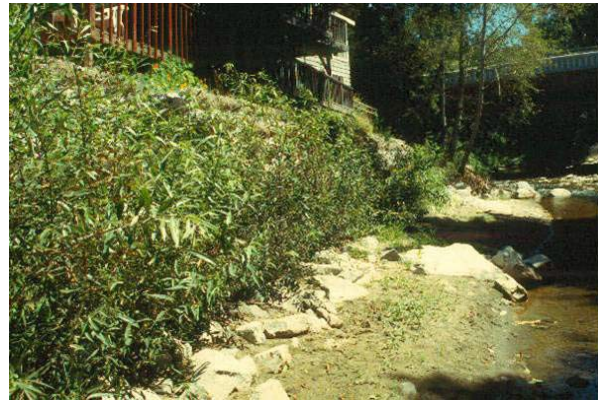
Photo 19. Brush Layering with soil warp used to stabilize a stream bank. Source: Salix Applied Earth Care
