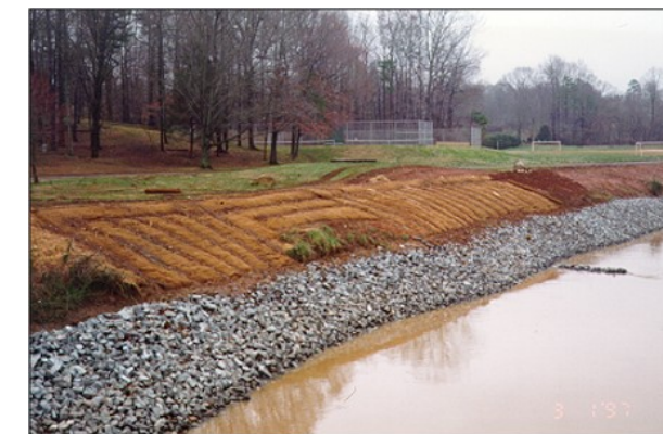
Photo 16. Fascines placed at angles and on contours. Source: Charlotte-Mecklenburg Storm Water Services
