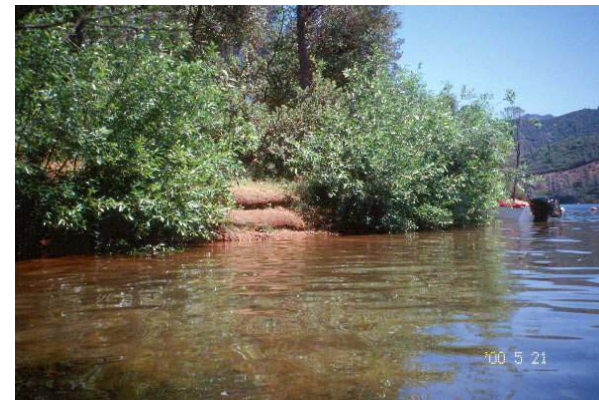
Photo 22. Brush layering, including soil warp, Whiskeytown Lake, CA. Source: Salix Applied Earth Care
