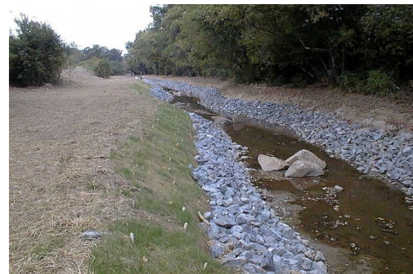
Photo 27. Erosion control matting with seed growing through. Source: Charlotte-Mecklenburg Storm Water Services
