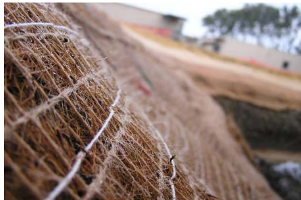
Photo 28. Erosion control matting. Source: Salix Applied Earthcare
