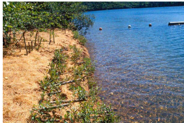
Photo 21. Brush layering, including soil warp, Whiskeytown Lake, CA. Source: Salix Applied Earth Care
