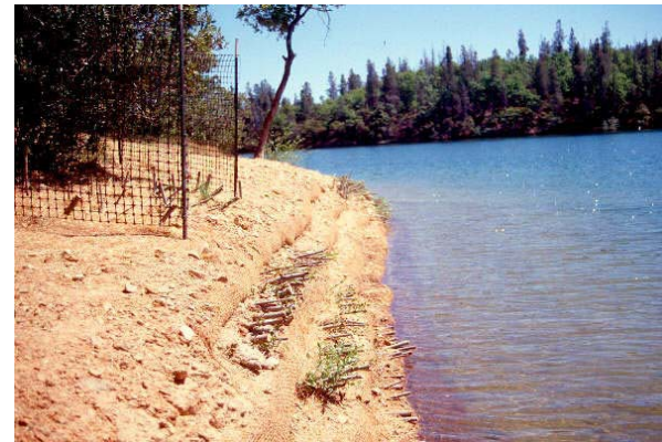
Photo 20. Brush layering, including soil warp, Whiskeytown Lake, CA. Source: Salix Applied Earth Care
