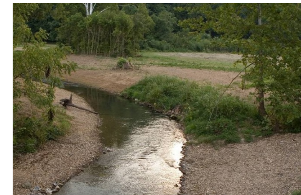
Photo 34. Sod matting on outside of a meander bend. Source: Stantec
