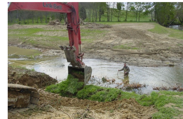
Photo 36. Excavator placing sod matting. Source: Bluegrass Streams, LLC
