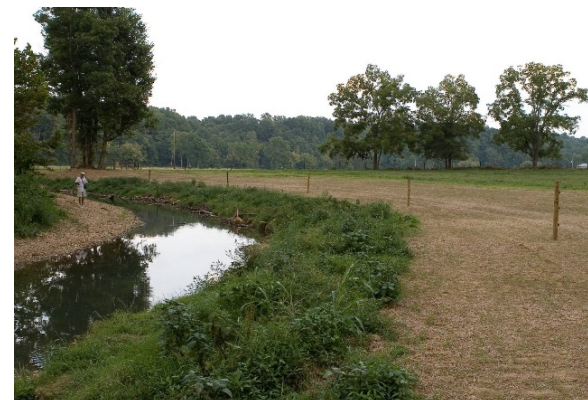
Photo 35. Sod matting on stream banks. Source: Stantec
