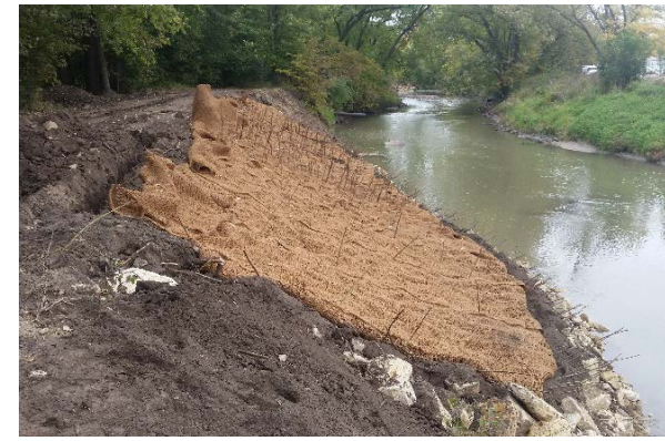
Photo 29. Erosion control matting installed on slope. Source: Iowa DNR
