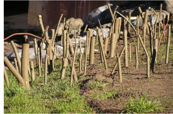
Photo 2. Installed live stakes prior to trimming. Source: Bio Draw-a product of Salix Applied Earth Care, 1996
