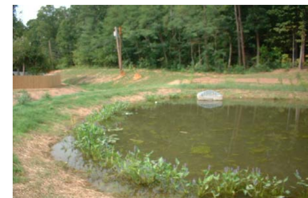
Photo 48. Vegetative plugs at Edwards Branch, NC. Source: Charlotte-Mecklenburg Storm Water Services
