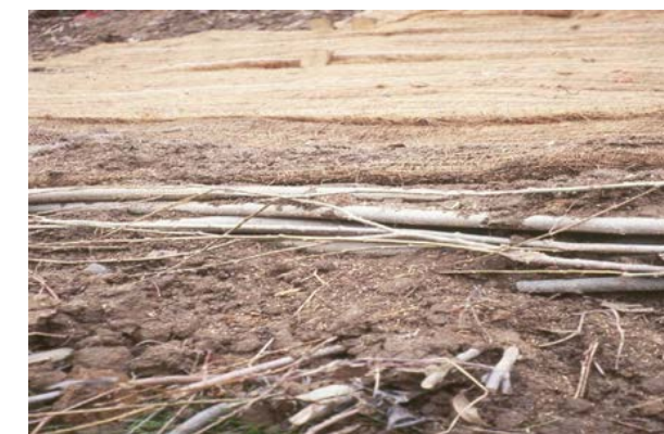
Photo 18. Installed fascine. Source: Stantec
