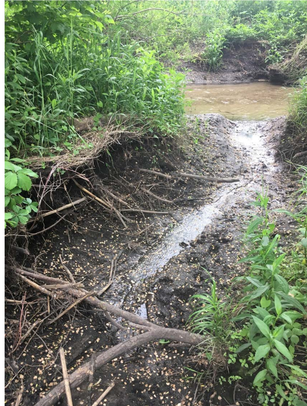
Figure 14. Gully erosion where edge of field drains into Dry Run.
