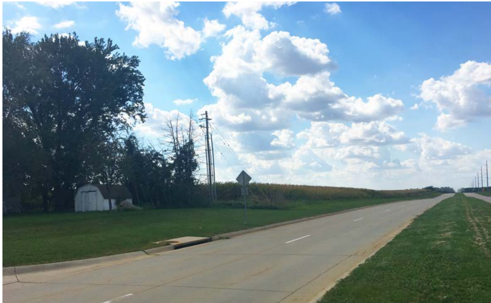
View along Ridgeway Ave facing West
