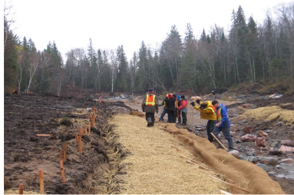
Photo 25. Top of slope trench for erosion control matting anchor. Source: Collins & Baker Engineering
