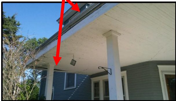
Damaged Porch Soffit and Fascia
