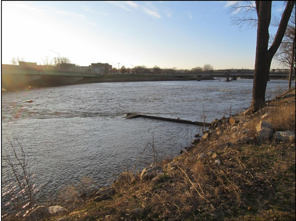
A view of the Clay Hole and remaining portion of the low head dam
