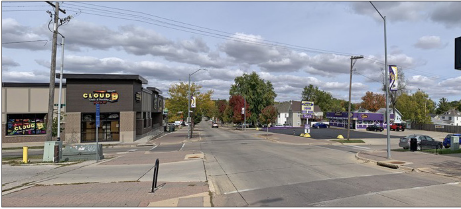
Existing conditions—College Street at 22nd Street, view to northeast
