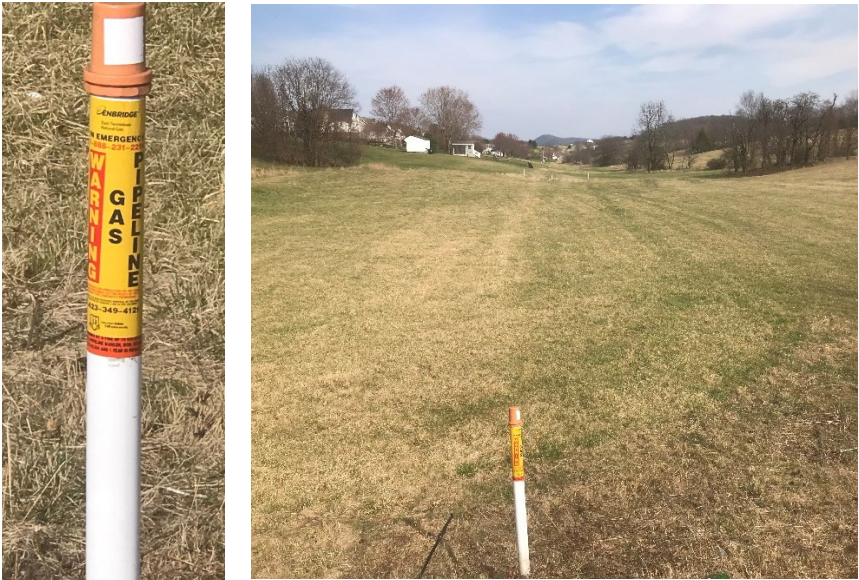
Images 6 and 7: Location of natural gas trunk line.
