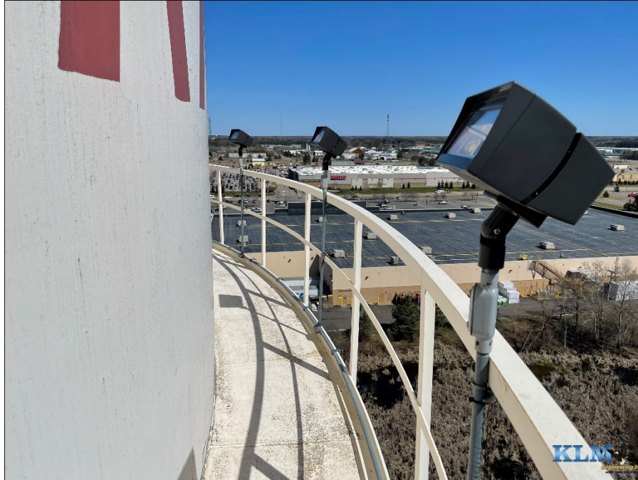
Photo No. 27 Balcony and handrail
