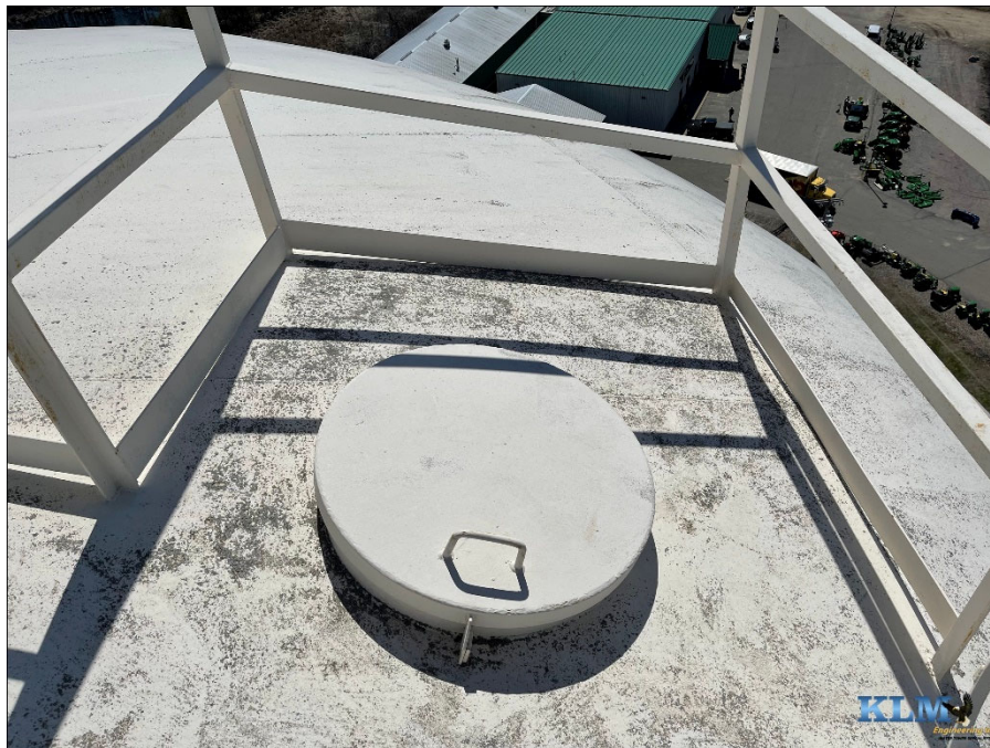
Photo No. 22 Wet access manway
