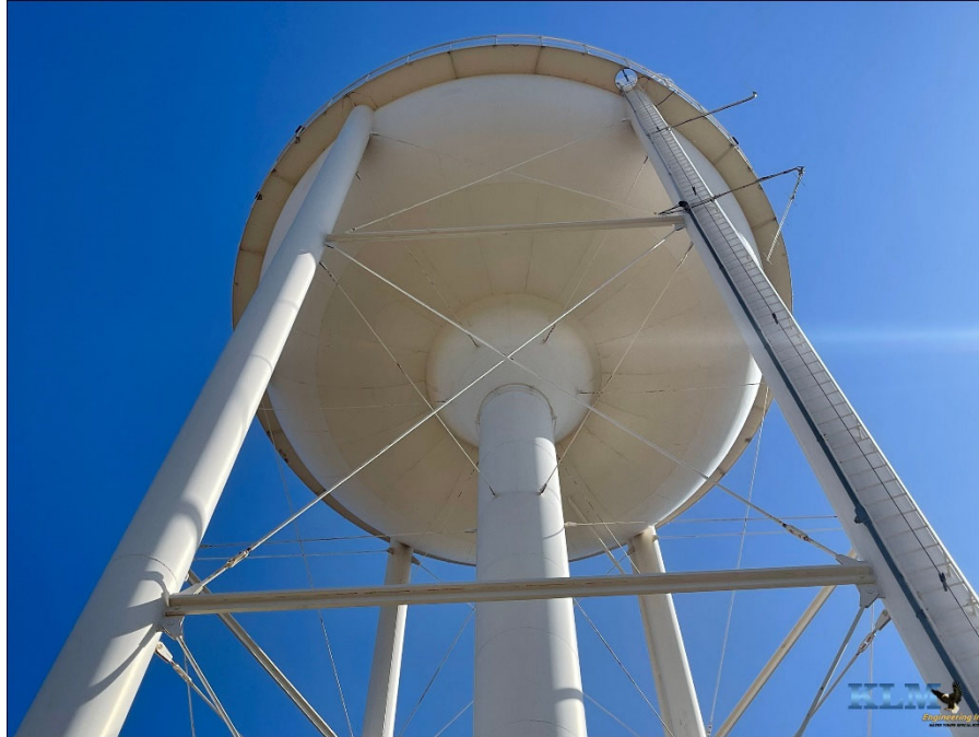
Photo No. 33 View of columns and wet riser
