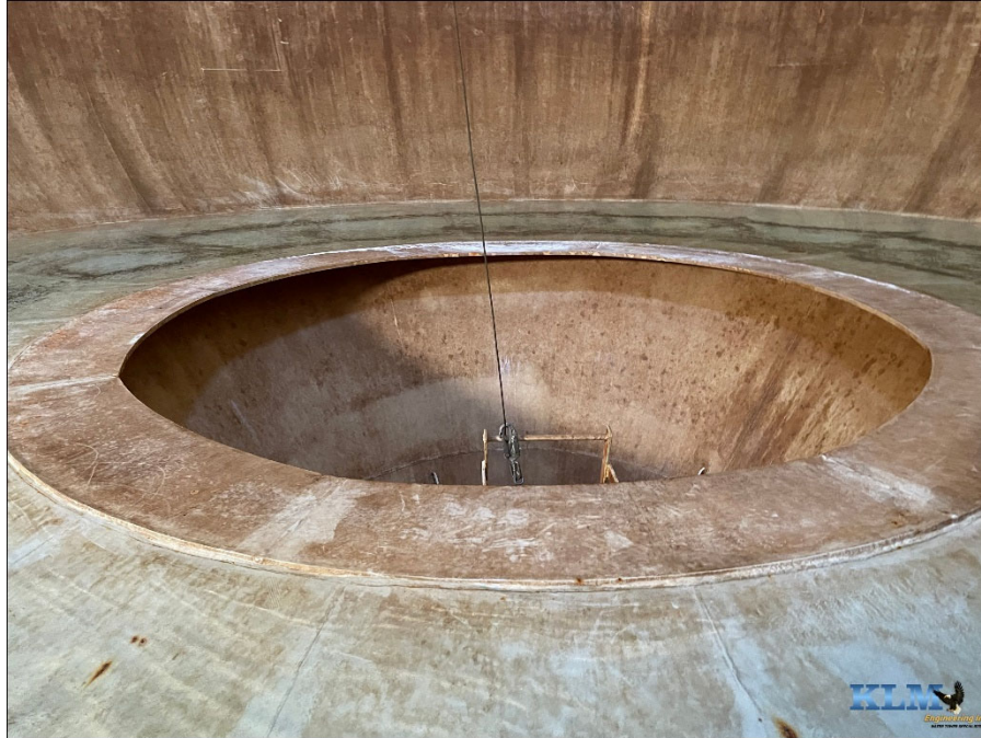
Photo No. 11 Top of cone
