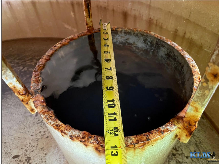
Photo No. 15 Condition of fill pipe
