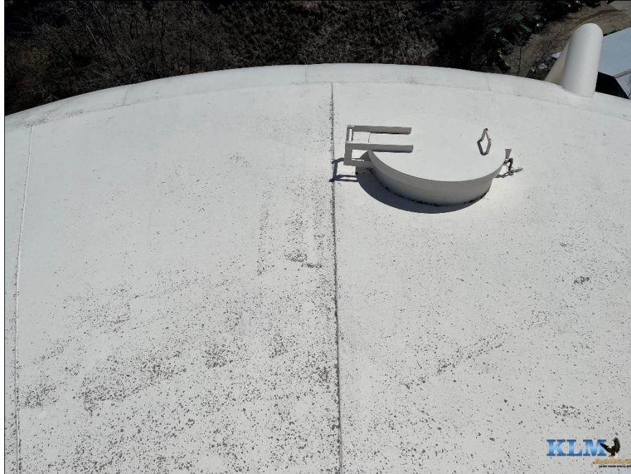
Photo No. 19 Roof plate coating conditions Ventilation manway visible
