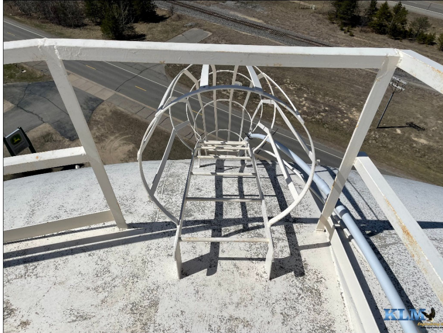
Photo No. 23 Roof access ladder
