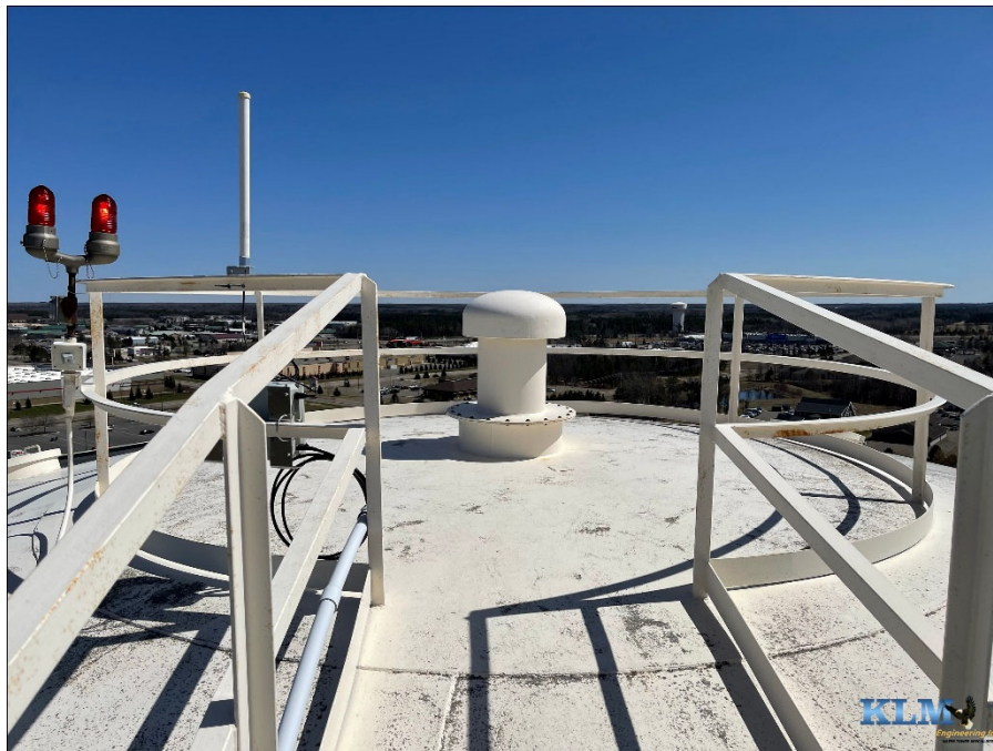
Photo No. 16 View of roof
