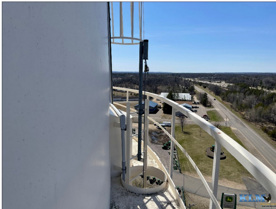
Photo No. 28 Balcony access
