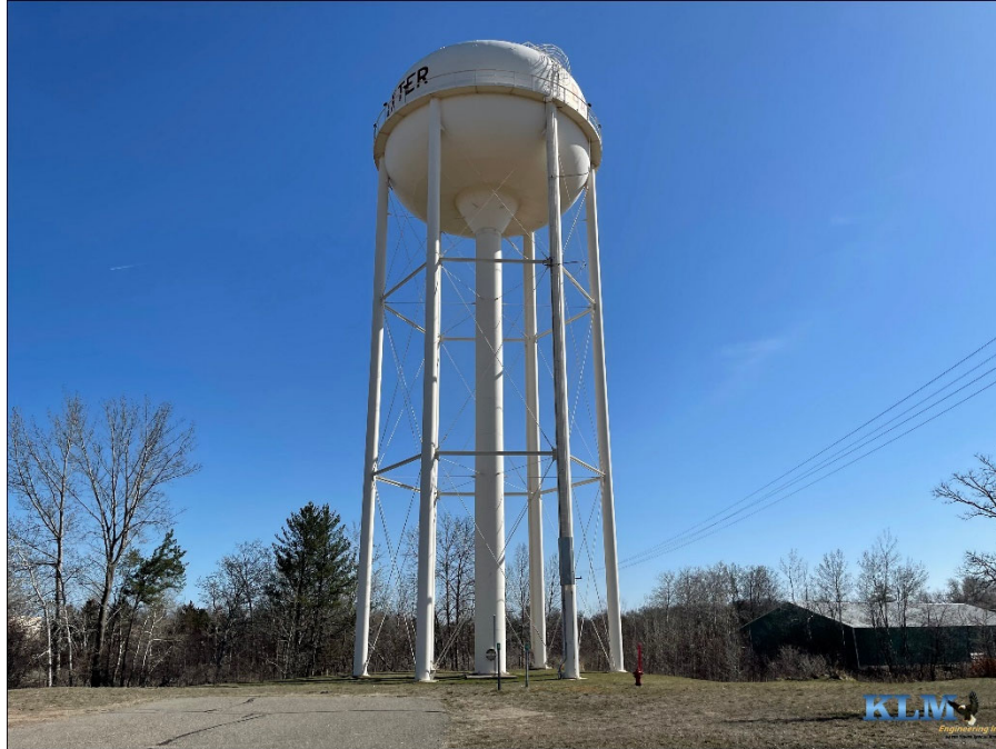
Photo No. 1 Overall view of the tower
