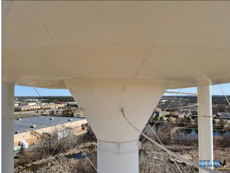
Photo No. 31 Bowl and cone coating conditions
