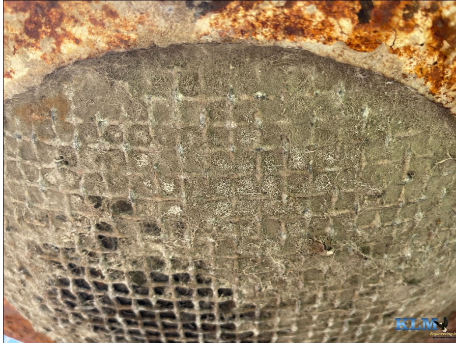
Photo No. 37 Condition of overflow pipe screen
