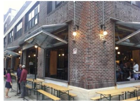
Example: Operable Windows and Overhead Doors
