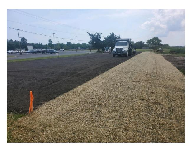
Re-establishing parking lot for Lenard Park with millings as a base, split-rail fence. Topsoil and seeding will be installed outside the parking area.
