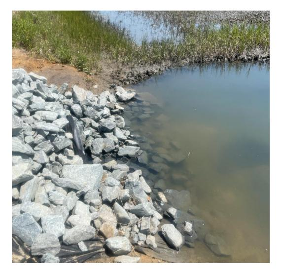
Rip Rap was installed to protect against erosion at both ends of each pipe.
