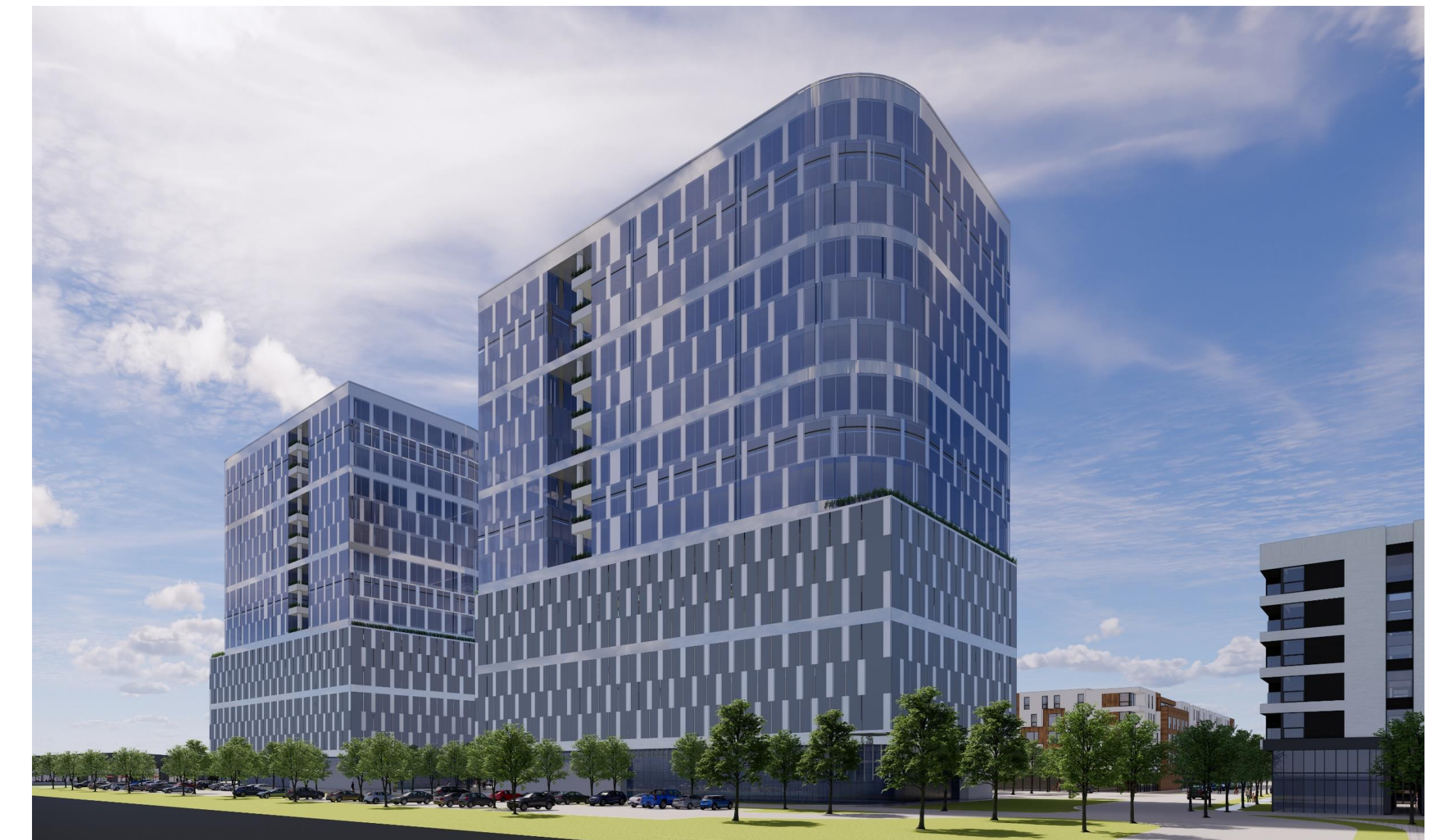
06 – OFFICE TOLLWAY VIEW
