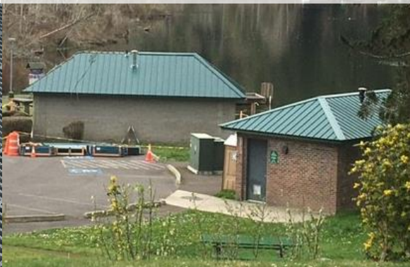
New Roof & ADA Fixtures Inside
