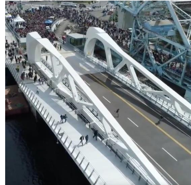
Johnson Street Bridge in Victoria (2018) features a 14 to 16 foot multimodal path on one side and a pedestrian-only pathway on the other.
